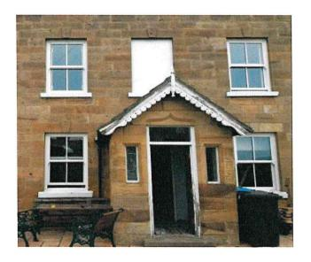
Below is the exiting opening to be replaced by a Victorian sash window of equal size and scale to the existing shown adjacent to the door opening. It is possible that the original opening was that of a window, it is clear that the stone lintel above the door is a replacement and would likely in our opinion have been replaced when the door opening was created.
