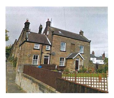
The porch entrance is utilised as the main entrance. The porch itself is an addition to the property, the stone coursing does not line through and the stone lintel detailing is more ornate and out of context with the original more simple Victorian style.
