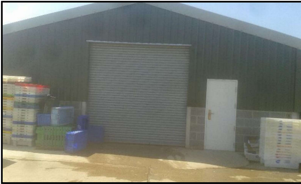
Photograph 4: Eastern elevation of building 3.
