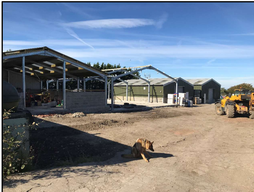
Photograph 1: View into the site from the existing access
