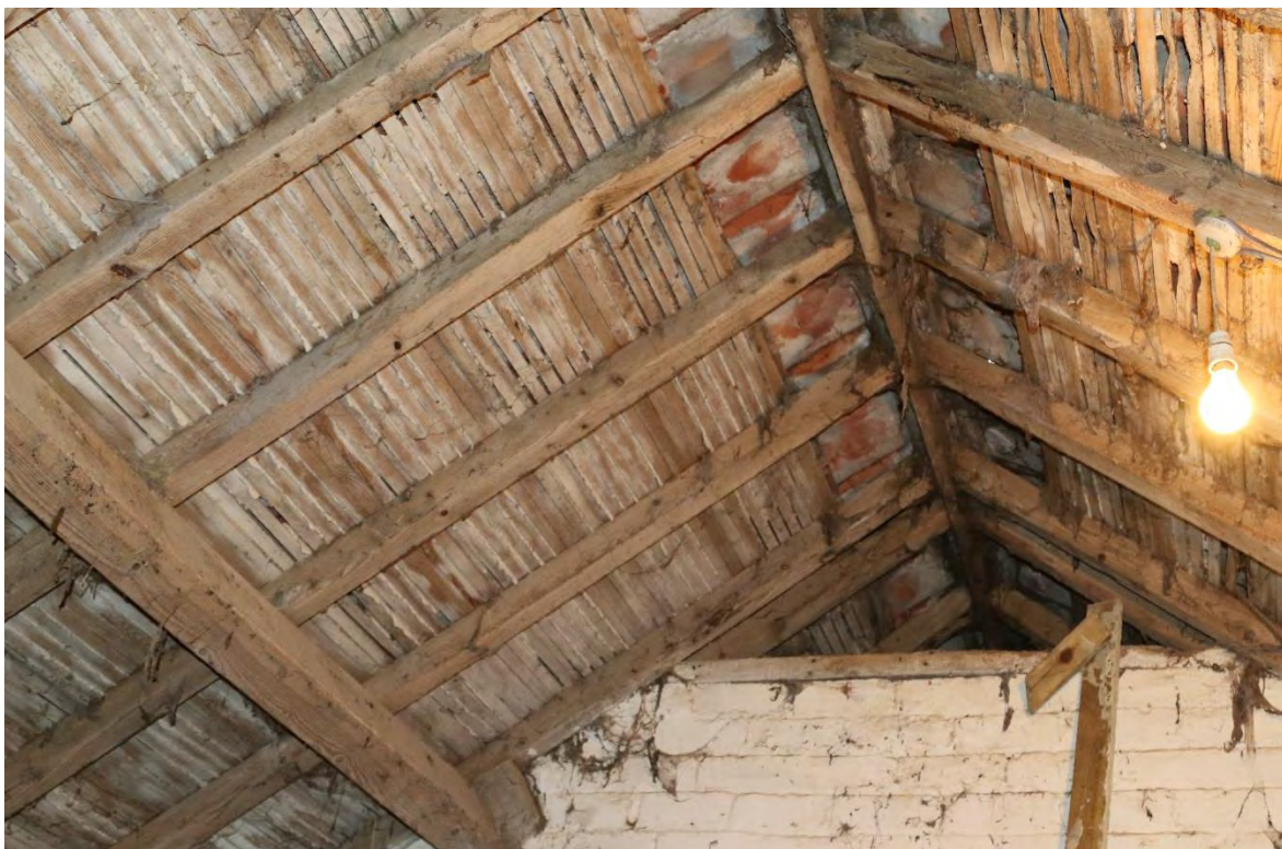
Image 8 – Further views from below the roof coverings within the building
