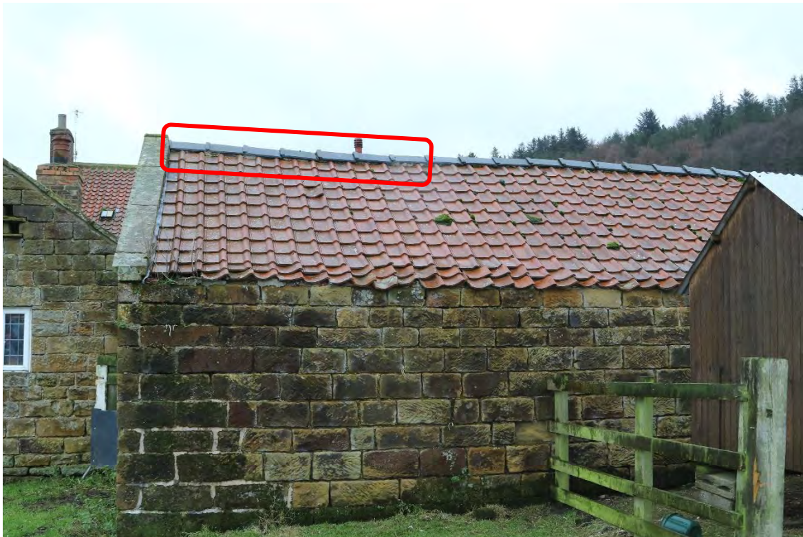
Image 5 – Movement noted within a number of ridge tiles which offer suitable roosting opportunities for crevice dwelling bats
