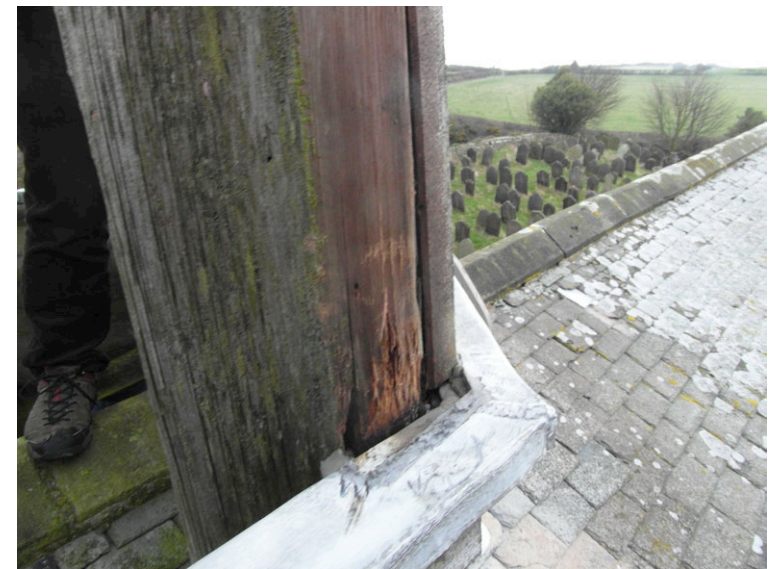
With the fascia removed decay can be seen in the post, a result of the water getting behind the fascia and not drying out.
