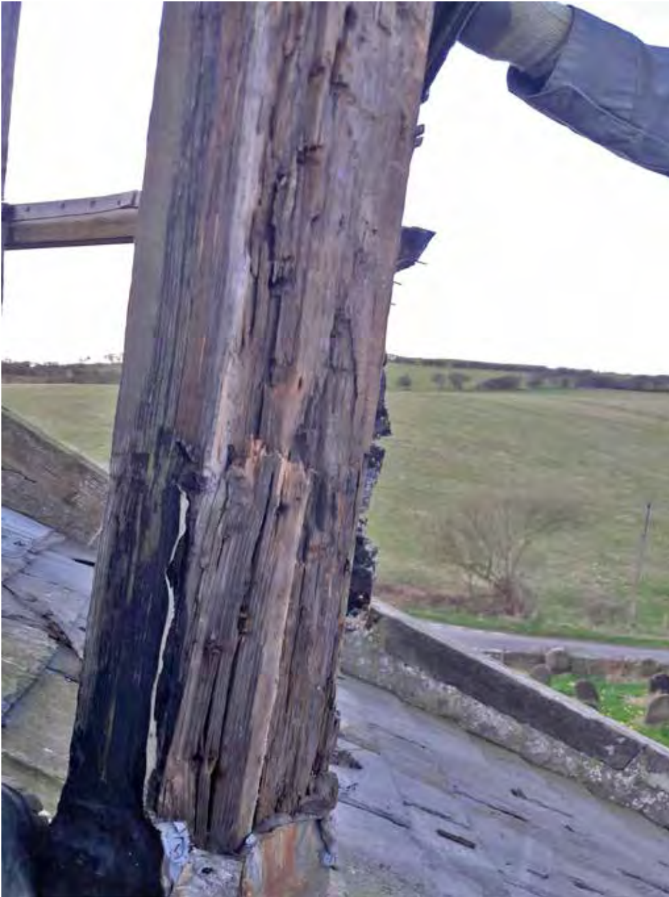
Decay in the timber was not helped by a lack of air movement preventing the posts to dry out.
