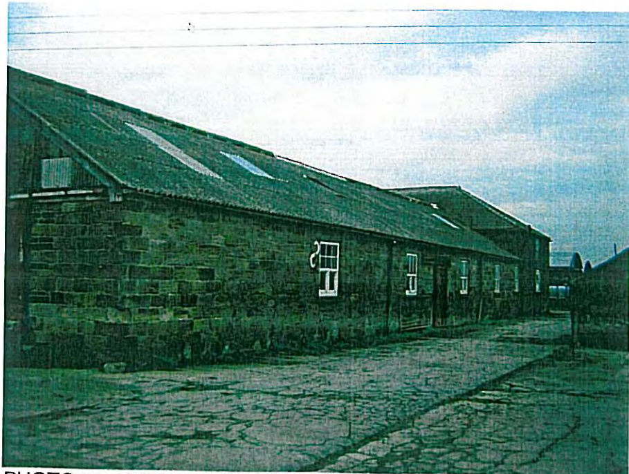
PHOTO 22. UNIT 7 – SIDE ELEVATION (3.08)
