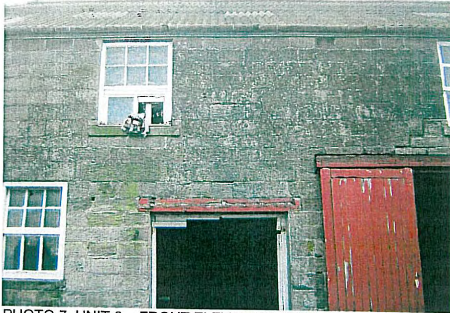
PHOTO 7. UNIT 3 – FRONT ELEVATION (3.03)
