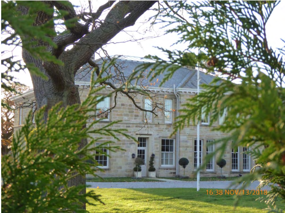
Figure 8: Views of the Listed property
