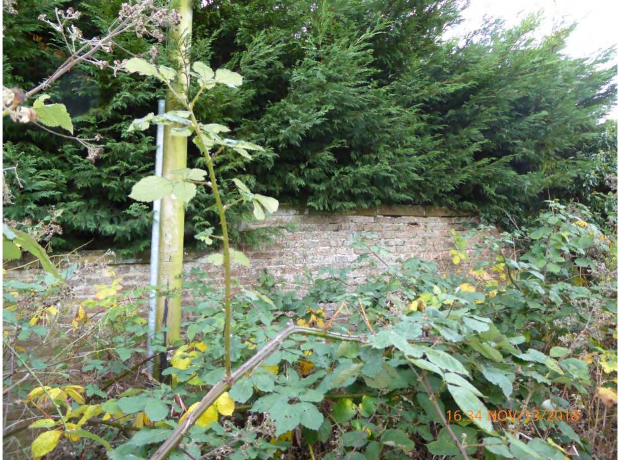
Figure 9: View of the Listed wall
