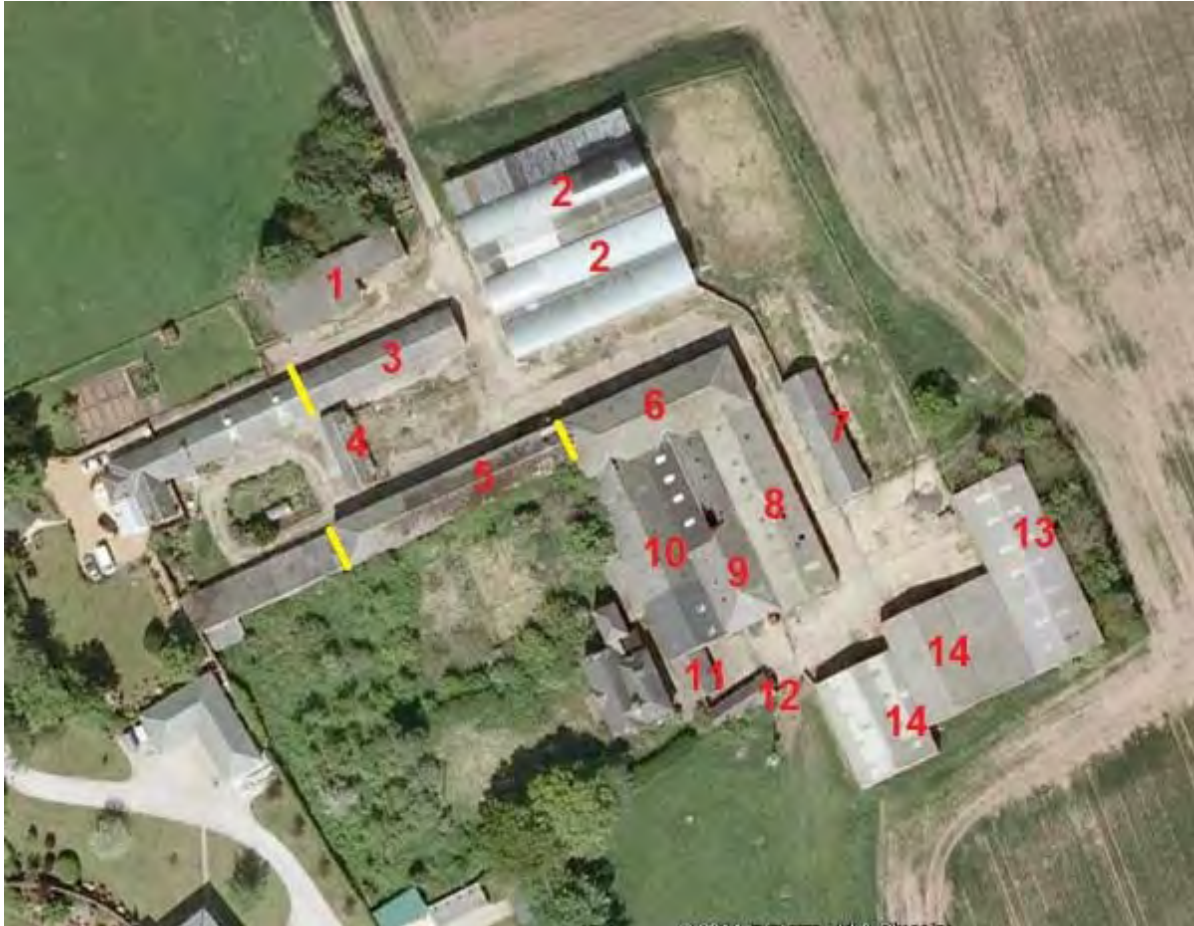
Figure 1 Building Numbers From Survey
