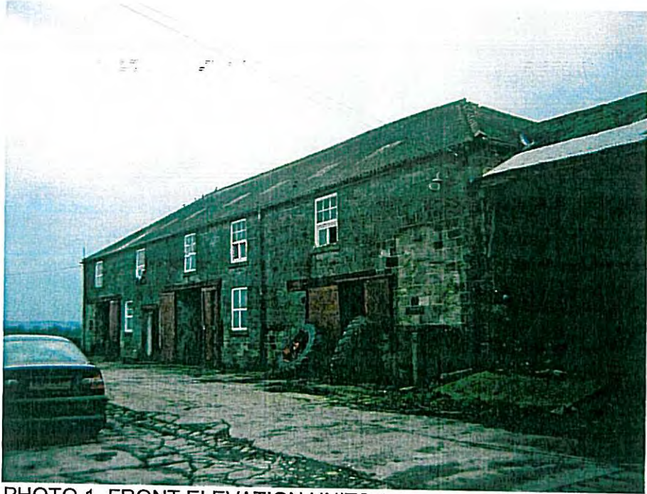
PHOTO 1. FRONT ELEVATION UNITS 1-4
