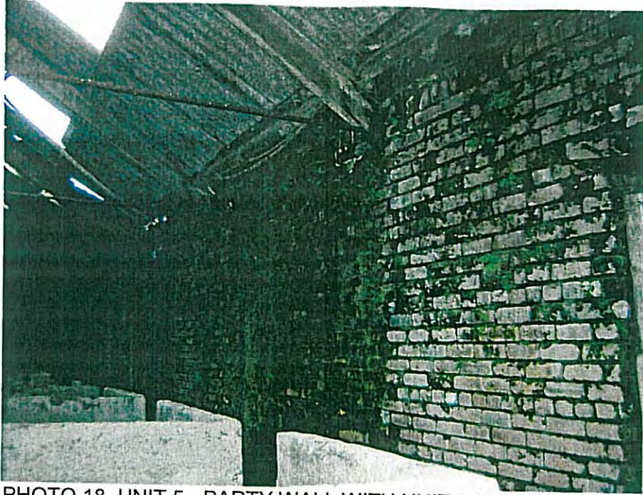
PHOTO 18. UNIT 5 - PARTY WALL WITH UNIT 6 (3.06.06)
