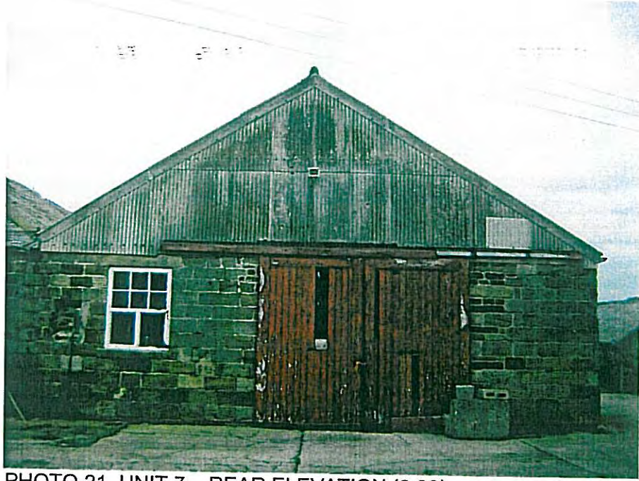
PHOTO 21. UNIT 7 – REAR ELEVATION (3.08)
