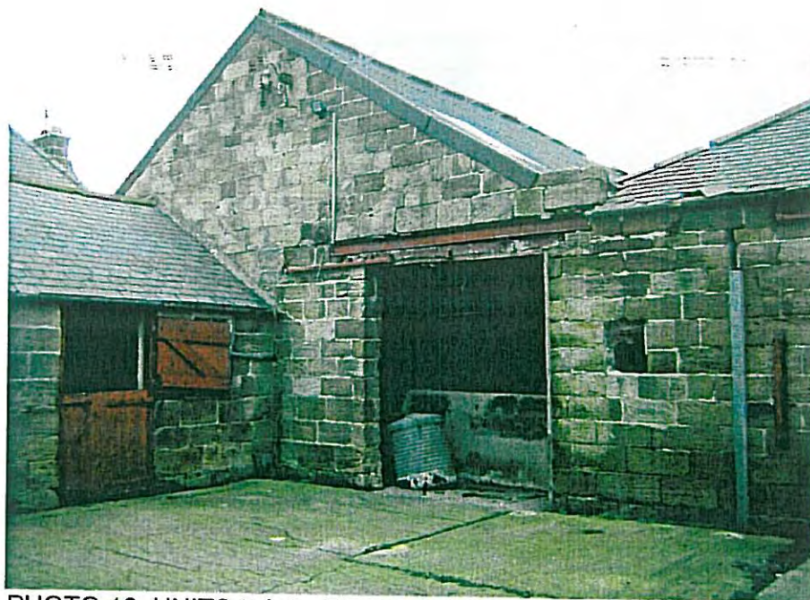
PHOTO 16. UNITS 5 & 8 - REAR ELEVATION (3.06, 3.09)
