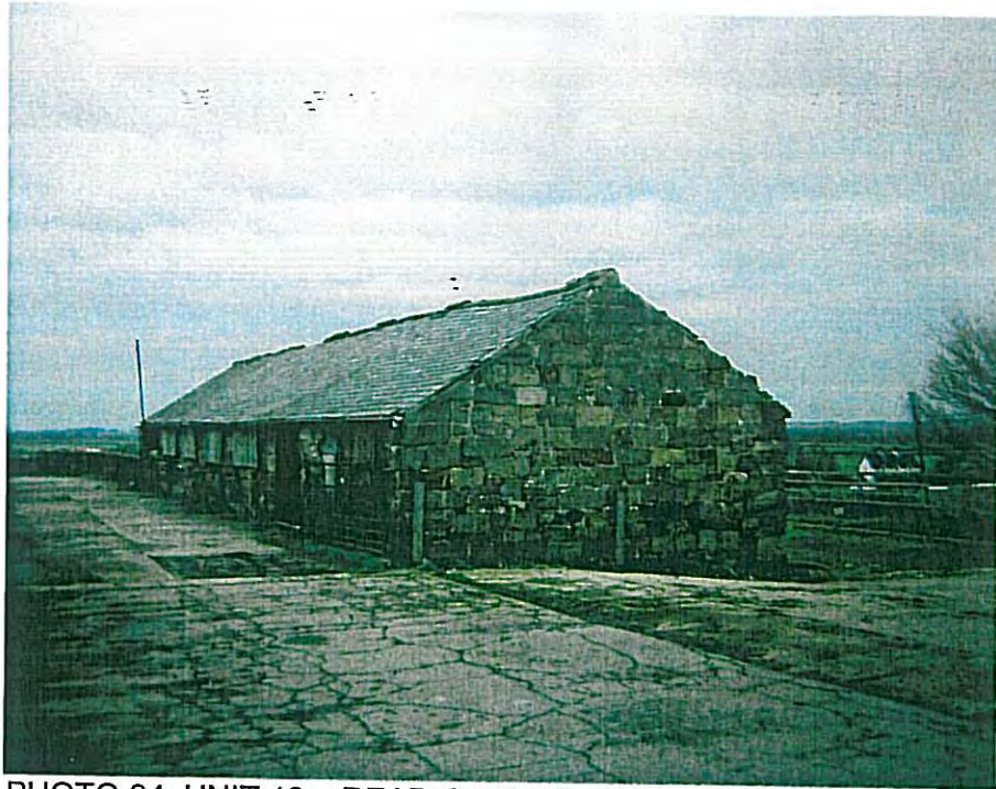
PHOTO 24. UNIT 10 – REAR GABLE & RIGHT HAND SIDE ELEVATION
