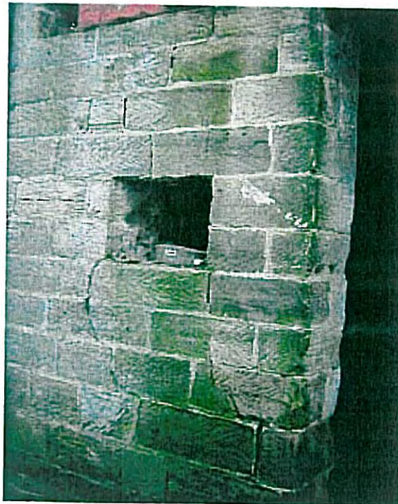
PHOTO 13. UNIT 4 – IMPACT DAMAGE (3.04.05)
