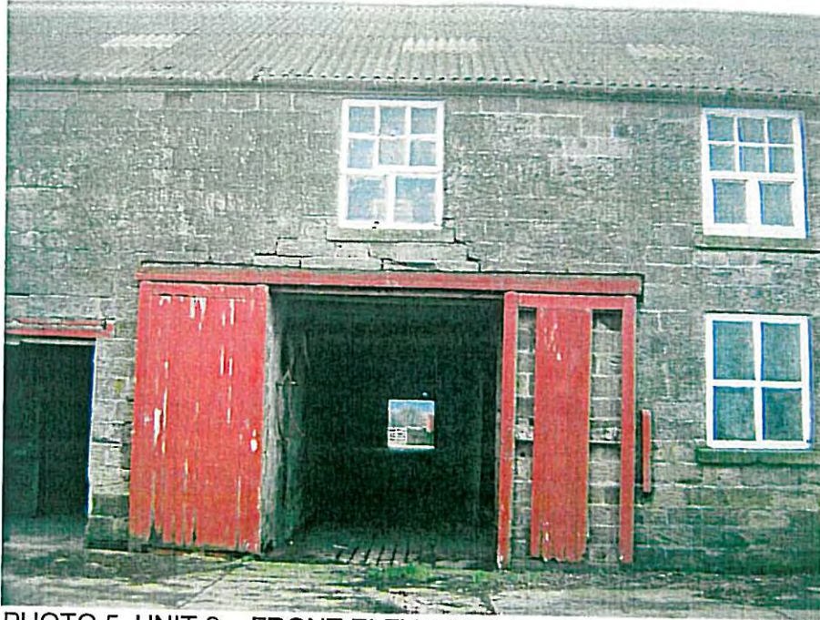
PHOTO 5. UNIT 2 – FRONT ELEVATION (3.02)
