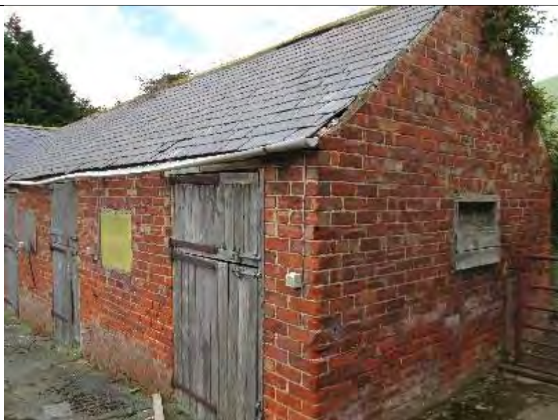
Building 4 south gable and west face.
