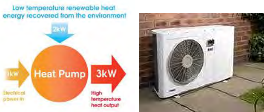
Fig. 3a & 3b: Air Source Heat Pump – Heat Pump Chart (left) & In-situ ASHP (right)
