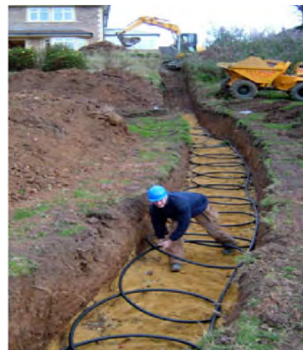
Fig. 4a & 4b: Ground Source Heat Pump – GSHP Typical System (left) & In-situ GSHP Slinky Pipe Run (right)
