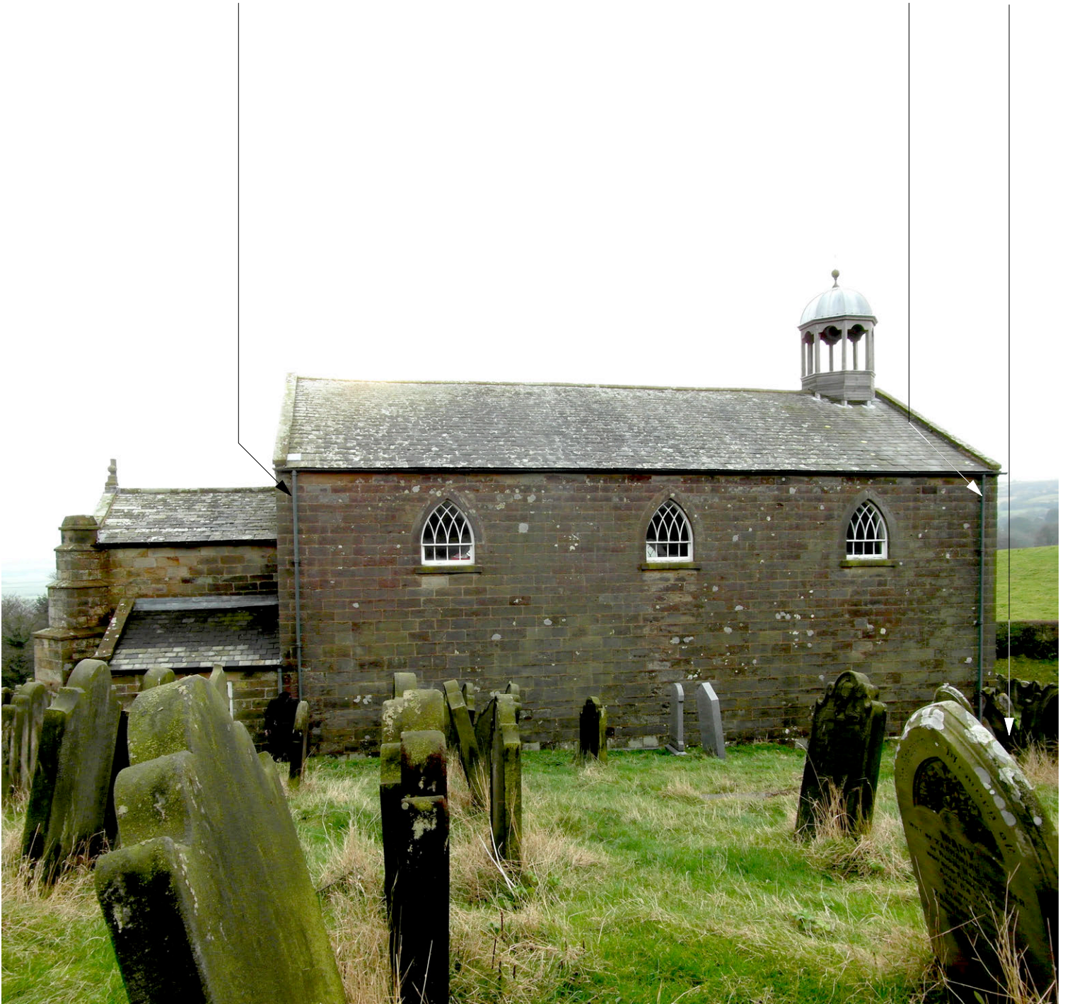
OLD ST STEPHENS CHURCH NORTH ELEVATION - EXISTING (before cupola boarding removed)
