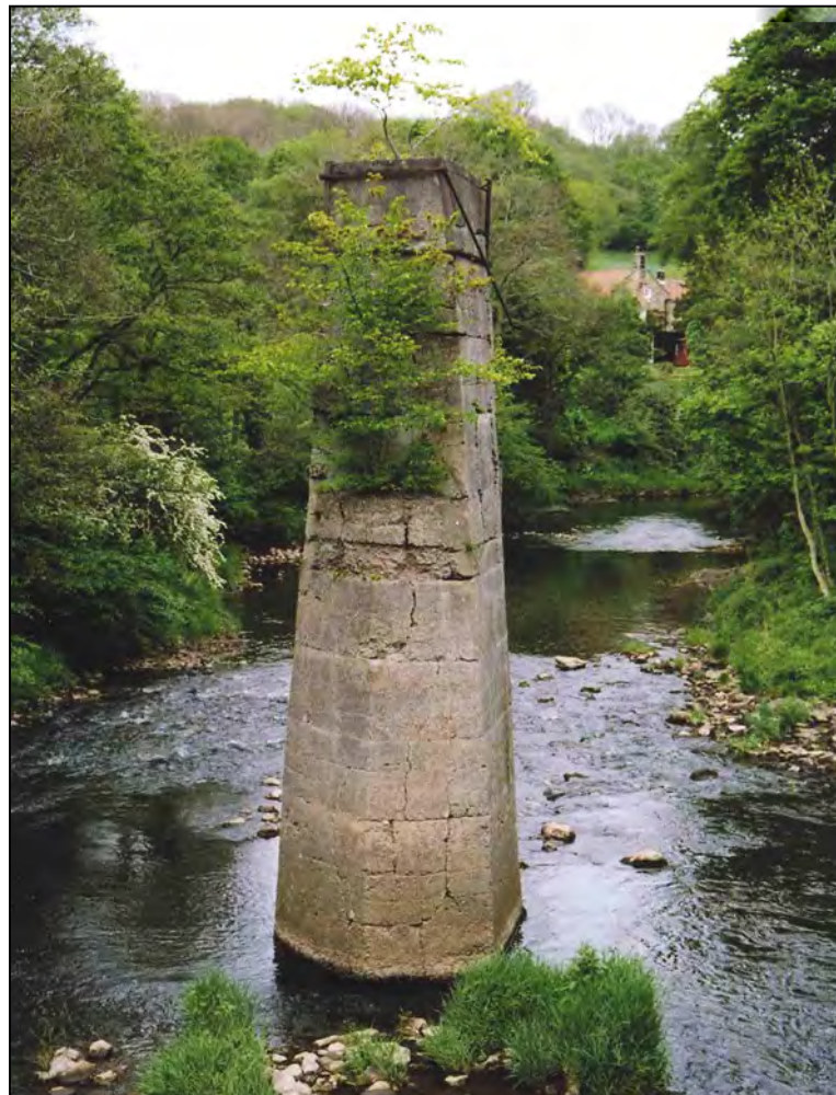
Plate 8: Bridge pier (part of Site 19), looking N.
