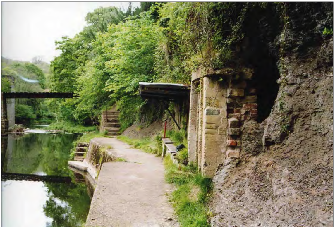
Plate 10: Wharf and related structures (Site 22), looking NE.
