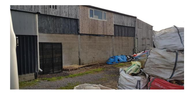
This photograph also shows the new timber window. A window did previously exist in this location. The previous window was formed by transparent plastic sheet behind timber cladding and provided limited light into the building.
