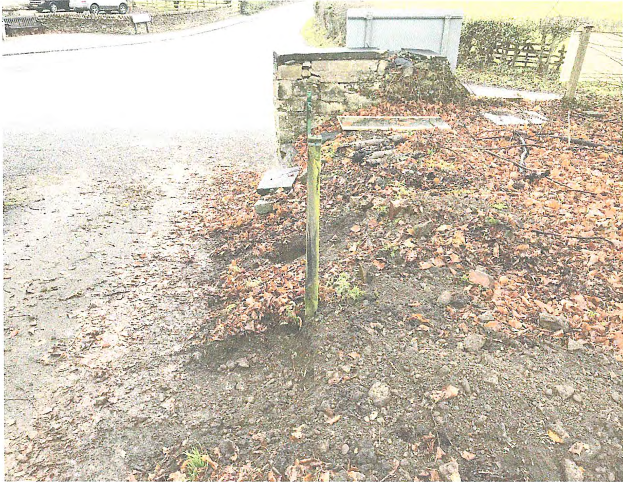
Photo 1 - Site entrance from inside the site
