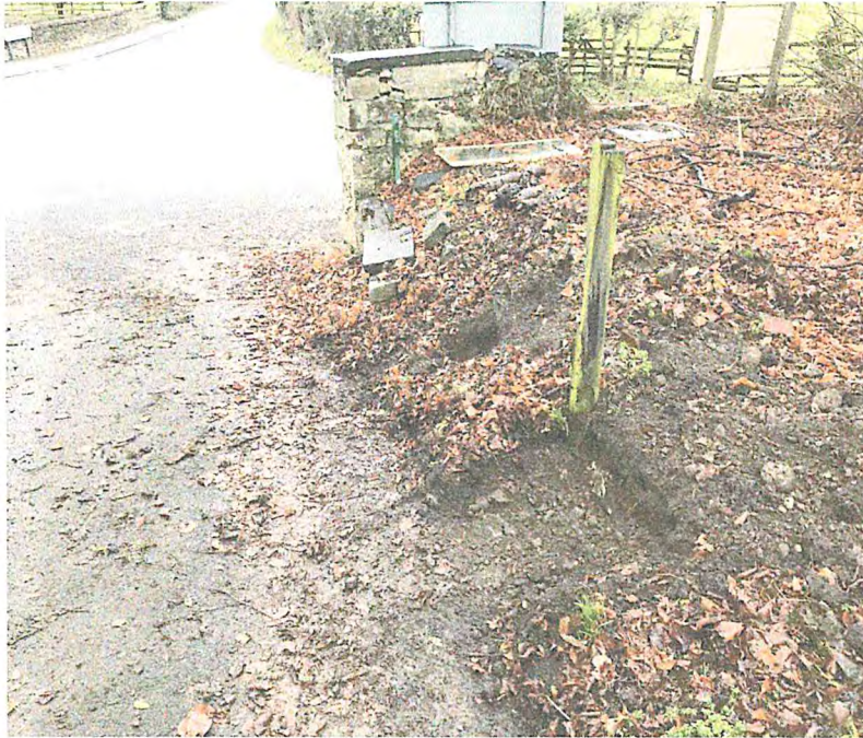
Photo 2 - General view of access driveway
