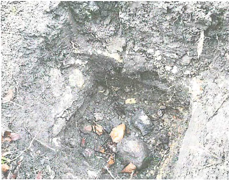
Photo 4 - Test excavation hole on access driveway
