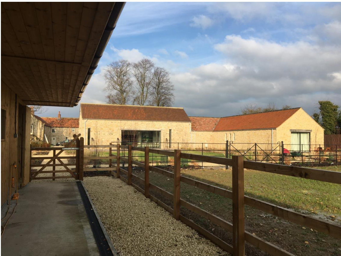
16 Fineline Aluminium Doors in Barn Conversion Context
