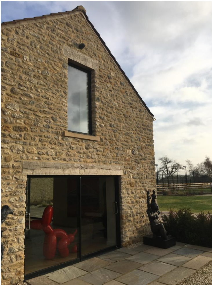
05 Smarts Systems Fixed Light Window to upper level, with Fineline Aluminium Sliding Door below (no comment re my Client's piece of "Art")
