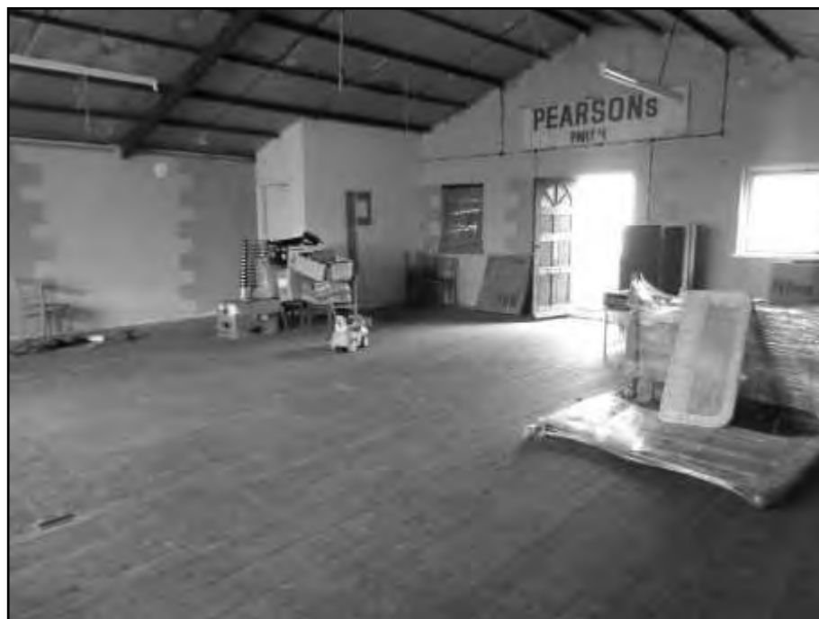
Figure 25. First floor open room (W.C. in far corner)
