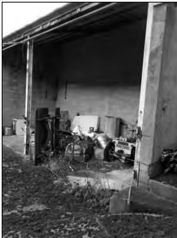
Figure 19. South eastern elevation with fascia board present
