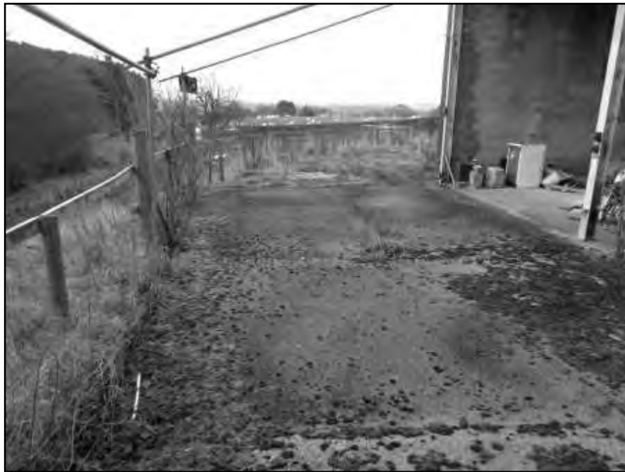
Figure 17. Hardstanding next to the south eastern elevation
