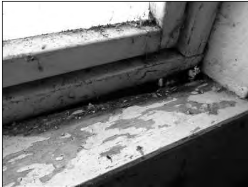
Figure 24. Example of first floor window sills
