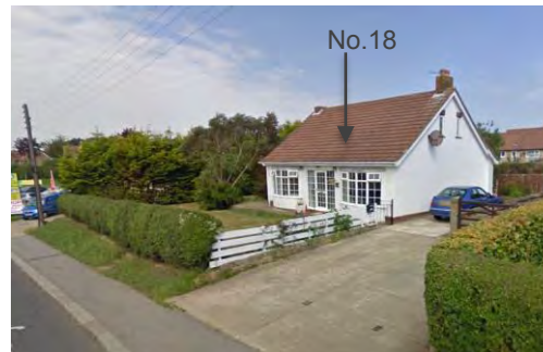
View to No.18 looking north west
