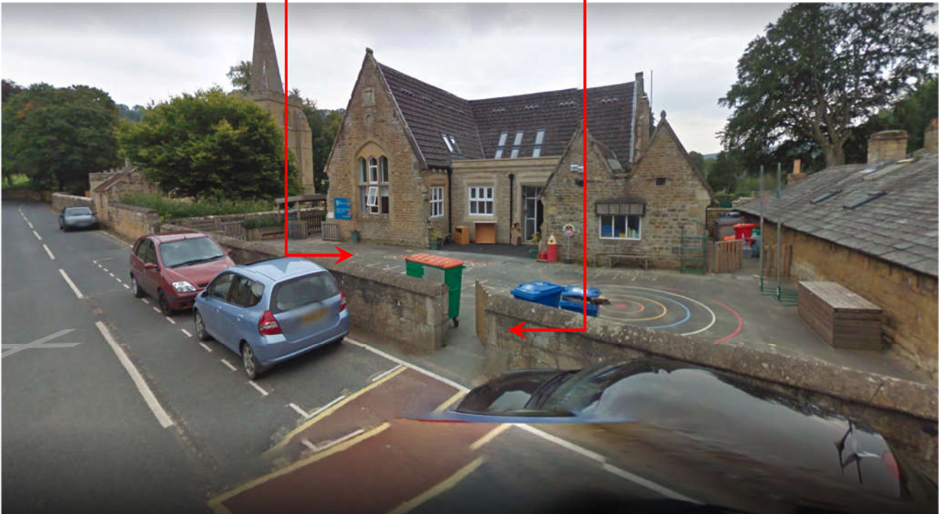
Figure 1 – North facing elevation. School playground and location of proposed new treatment plant.
