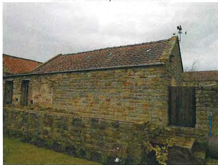
Plate 6 – Barn 2, south elevation.
