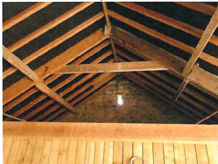
Plate 11 – Barn 2, internal roof structure
