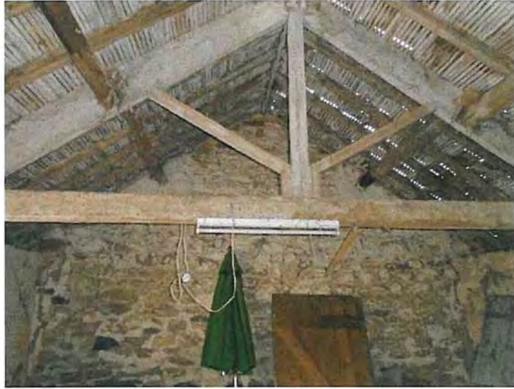
Plate 4 – Barn 1, internal roof structure.
