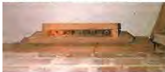
Plate 12 - Example of an open bottomed slot box (Norfolk Bat Group)
