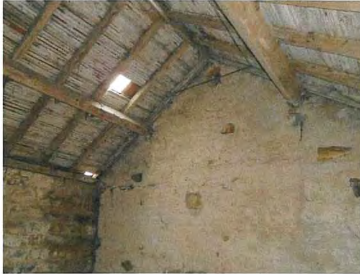
Plate 7 – Barn 2, internal roof structure
