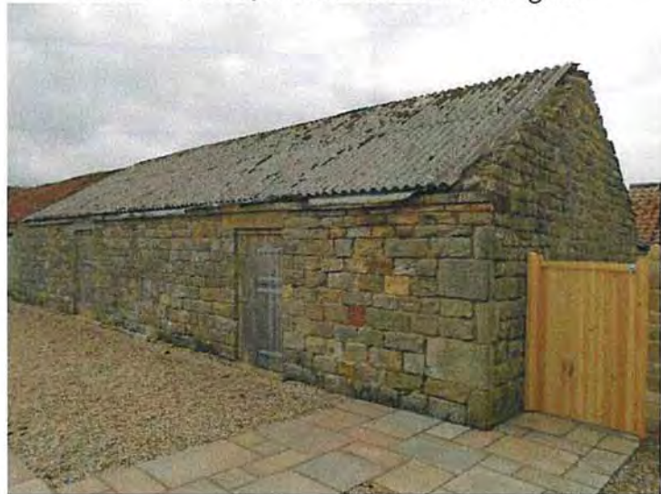
Plate 2 – Barn 1, east elevation and north gable.
