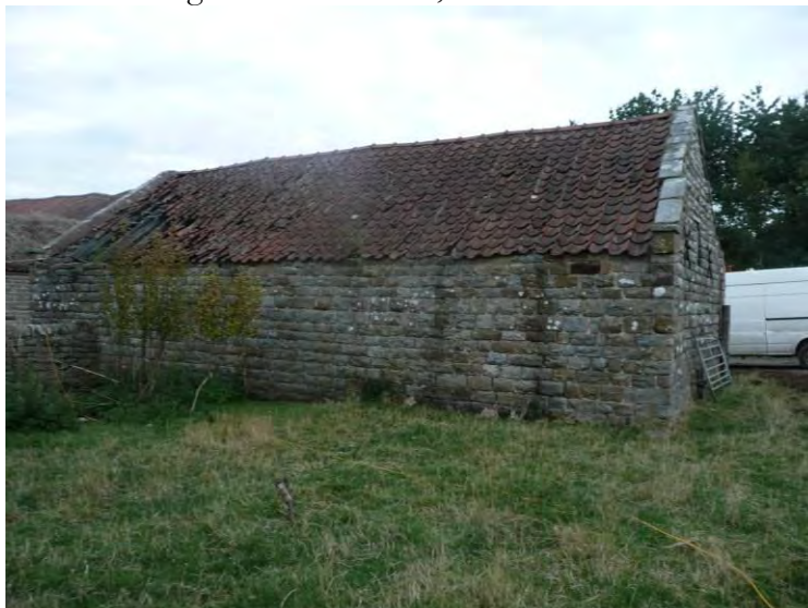
Figure 3 – Cart shed, south elevation.
