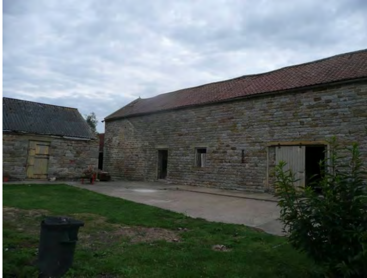
Figure 1 – Barn, south elevation.
