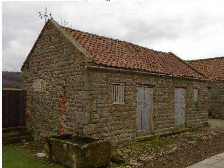
Plate 5 – Barn 2, east gable and north elevation.
