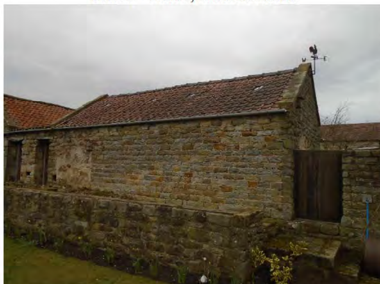
Plate 6 – Barn 2, south elevation.
