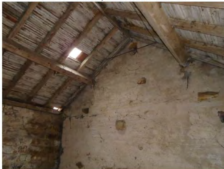
Plate 7 – Barn 2, internal roof structure
