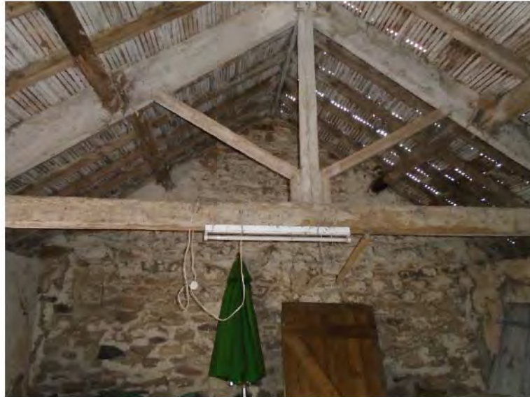
Plate 4 – Barn 1, internal roof structure.
