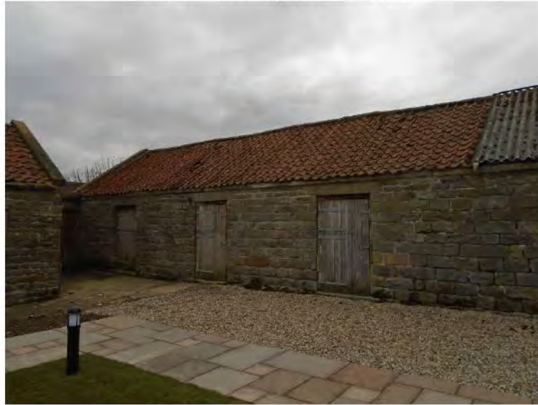
Plate 1 – Barn 1, east elevation.
