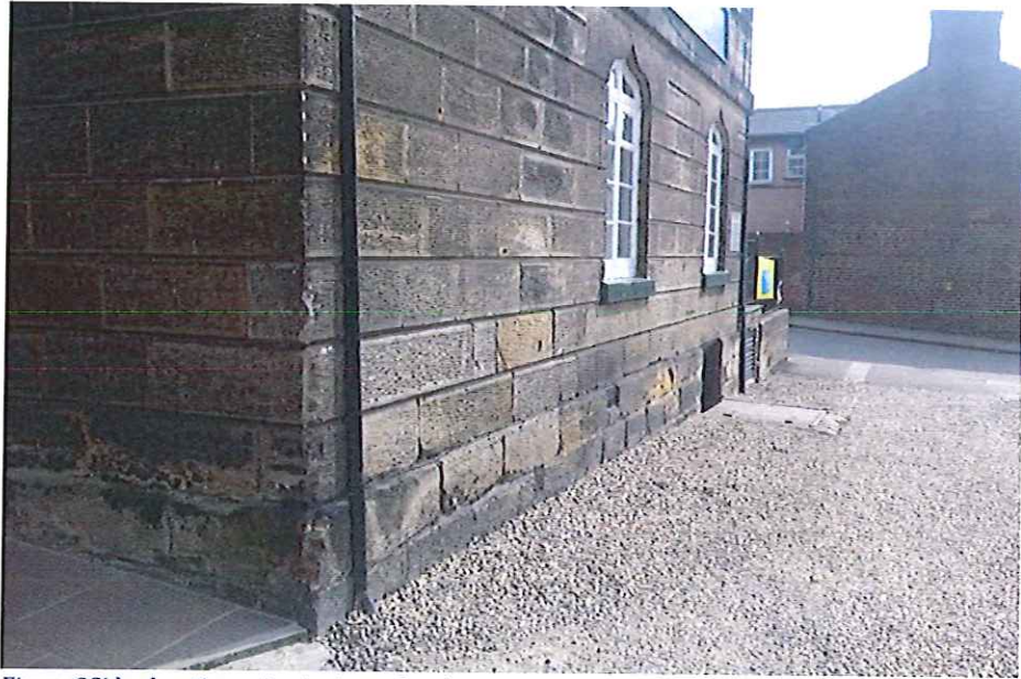
Figure 2 Side elevation prior to stone cleaning.
