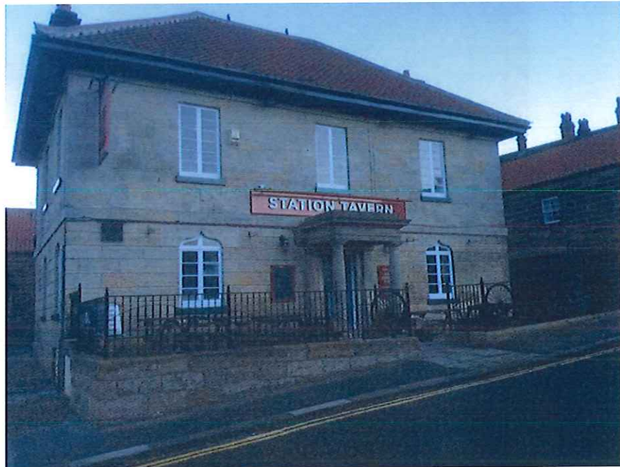
Figure 4 Front elevation after stone cleaning.
