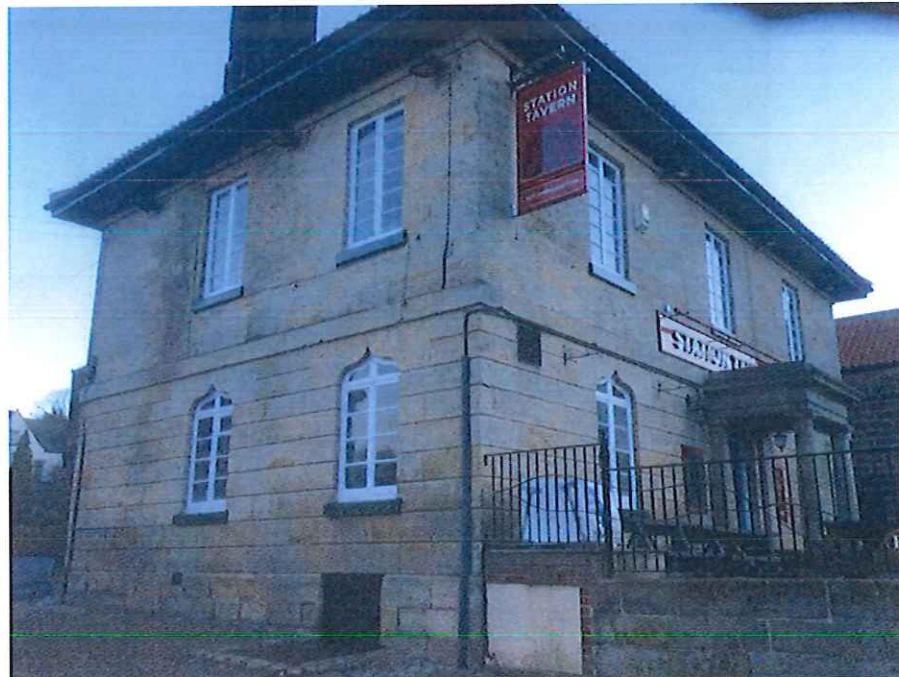
Figure 5 Side elevation after stone cleaning.
