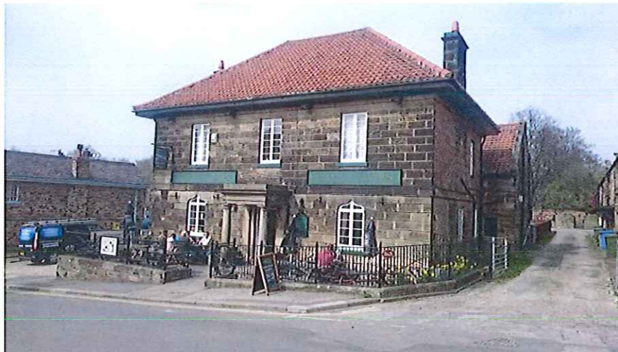
Figure 1 Building prior to stone cleaning front elevation.
