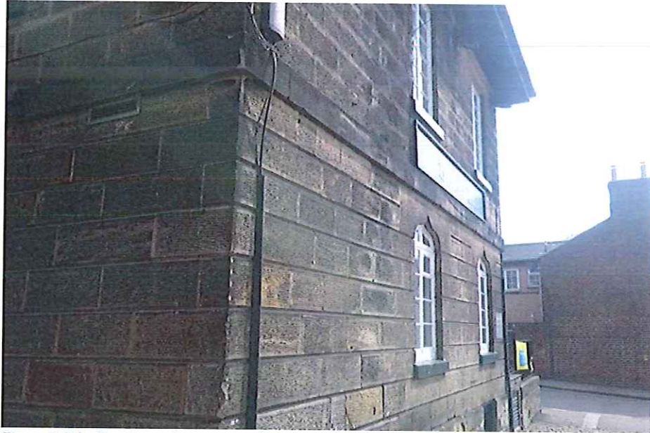
Figure 3 Side elevation prior to stone cleaning.
