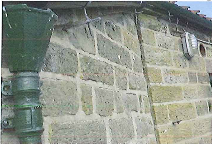
Photo 23: Walls and guttering
