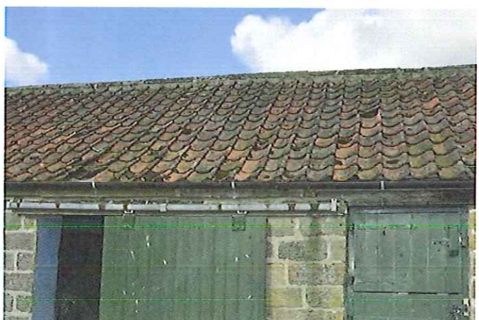
Photo 22: Roof of adjoining stores
