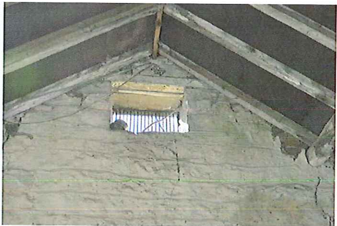
Photo 13: Aperture in gable end wall with close gapped grill.
