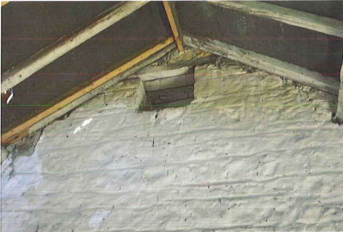
Photo 14: Opening through internal wall
