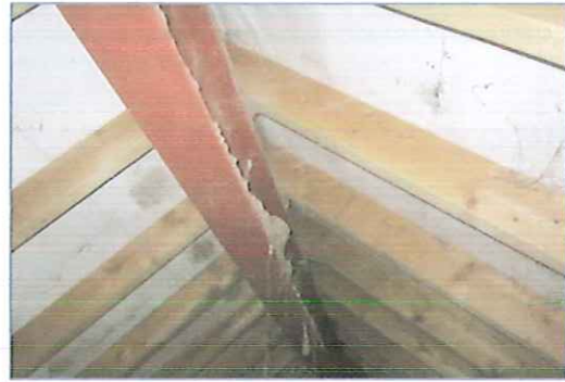
Photo 4 - Lined roof and steel beam with swallows nesting along beam.
