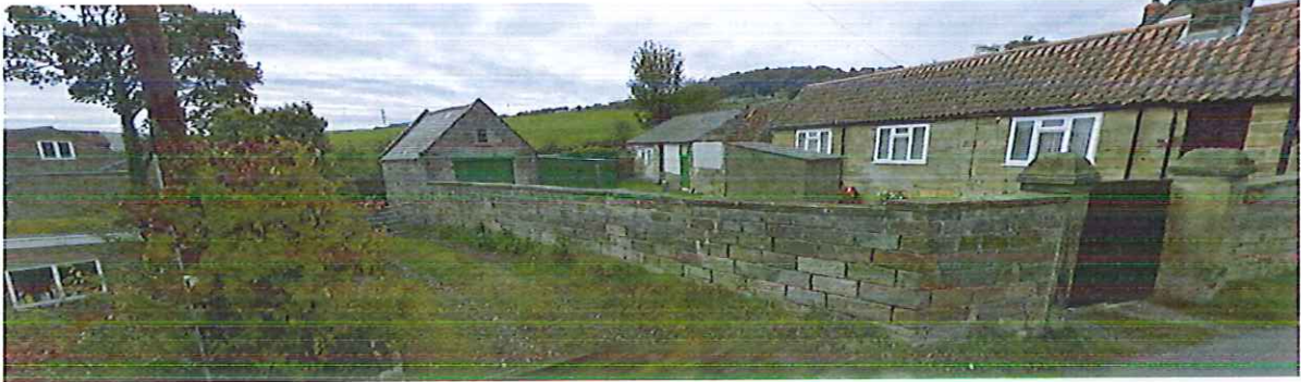
Examples of solid, masonry outbuildings throughout the Conservation Area
