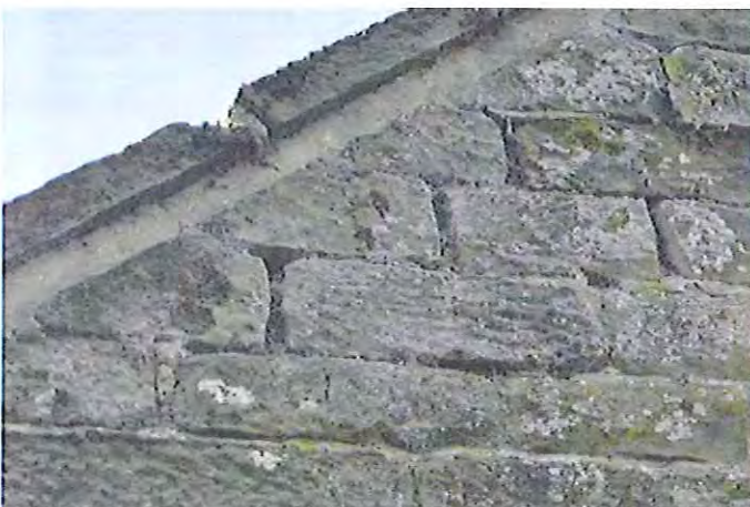
Photo 7 and 8: Cracks and holes in gable end wall.
