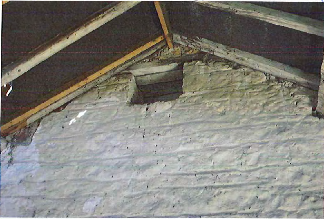
Photo 13: Opening through internal wall
