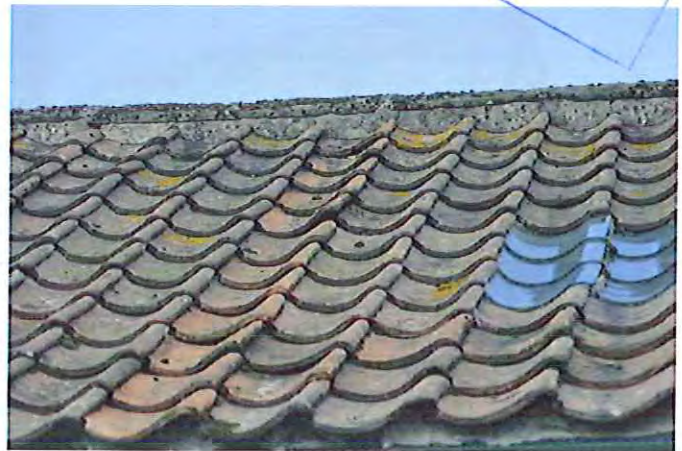
Photos 3 and 4: Photos of roof showing some raised and broken tiles, but intact ridge tiles and pointing.
