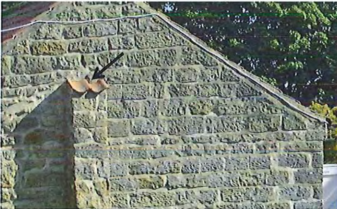
Photo 27: Gable end wall showing buttress topped with two pan tiles
