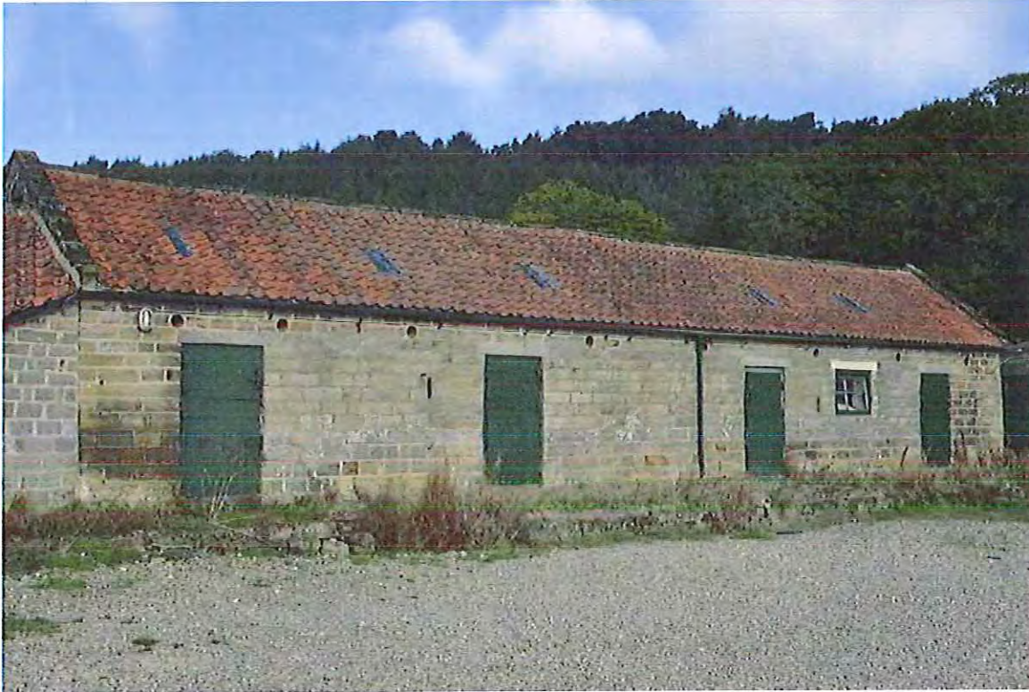
Photo 1: Disused Stable Block/Cow Byre
