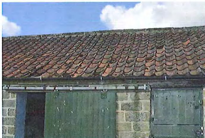
Photo 20: Roof of adjoining stores
