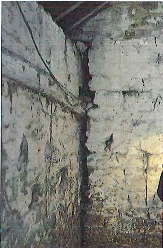
Photo 14 and 15 Cracks between internal and external walls.
