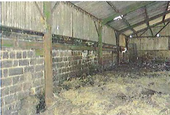
Photo 11: Rear wall of stable block.
