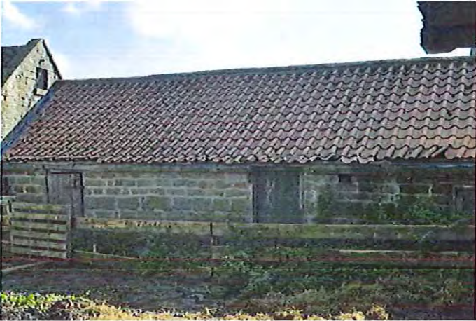
Photo 22: Rear Wall of adjoining stores.
