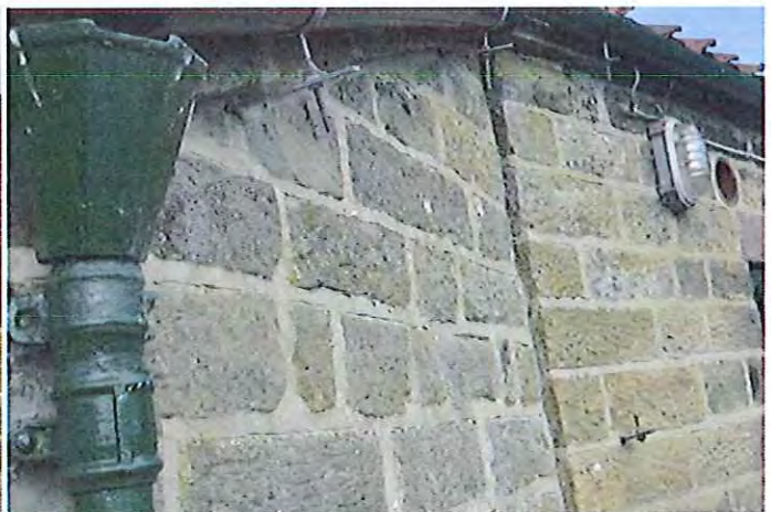
Photo 21: Walls and guttering
