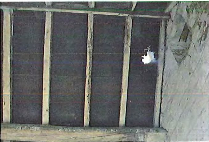
Photo 18: Hole in sarking and aperture through to adjacent room.
