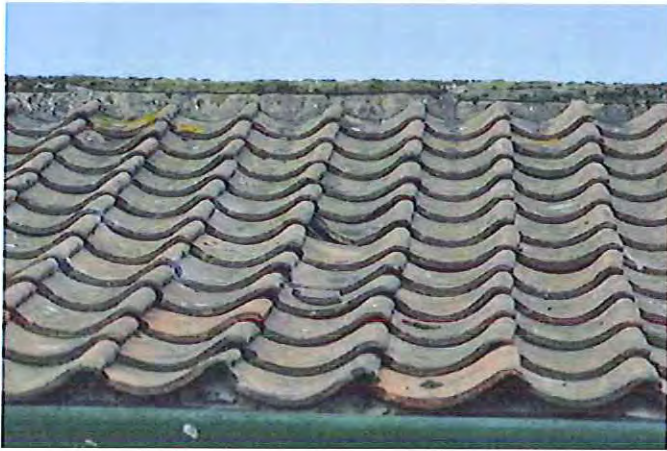
Photos 3 and 4: Photos of roof showing some raised and broken tiles, but intact ridge tiles and pointing.
