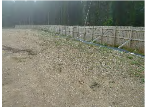
Photo 8: Southern boundary of the Site
