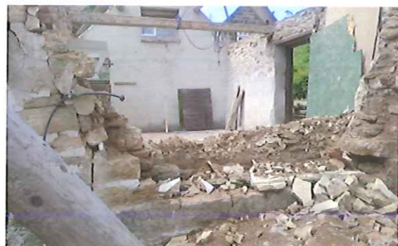
Earth and rubble filled walls
