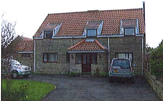
Existing building viewed from the North and Main Road
