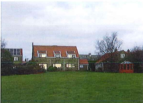
Existing building viewed from the South and the garden
