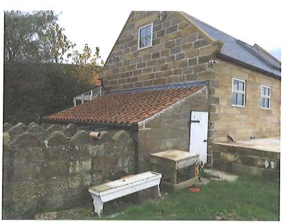
Gutter brackets could not be used as the wall is only a single skin wall and a proportion of the wall is taken up with door ways, so we regarded the replacement a repair.
