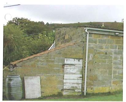
2) With regard to fascia on the north eastern elevation of outbuilding C, as you will see from the photo below, on the small lean to building (disused pig sty's), the rain gutter runs into a water butt, which then overflowed on to the grass, This gutter was mounted on a fascia board
