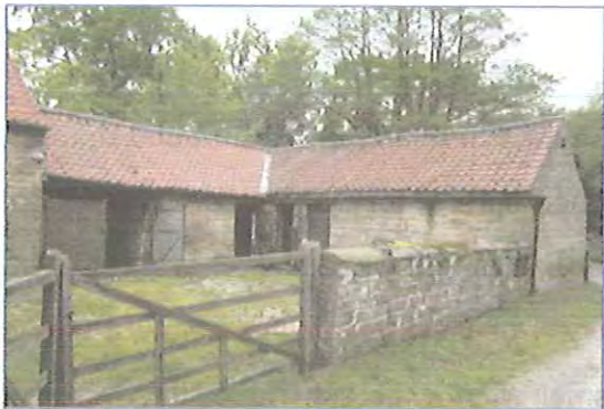
Photo 1 - View of the building from the courtyard (west).
