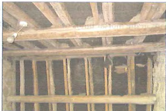
Photo 4 - Roof structure to unit a, showing old swallow nests on timbers.
