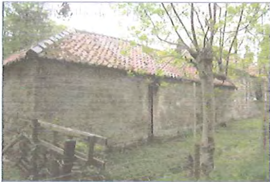
Photo 3 - Rear roof pitch (north).
