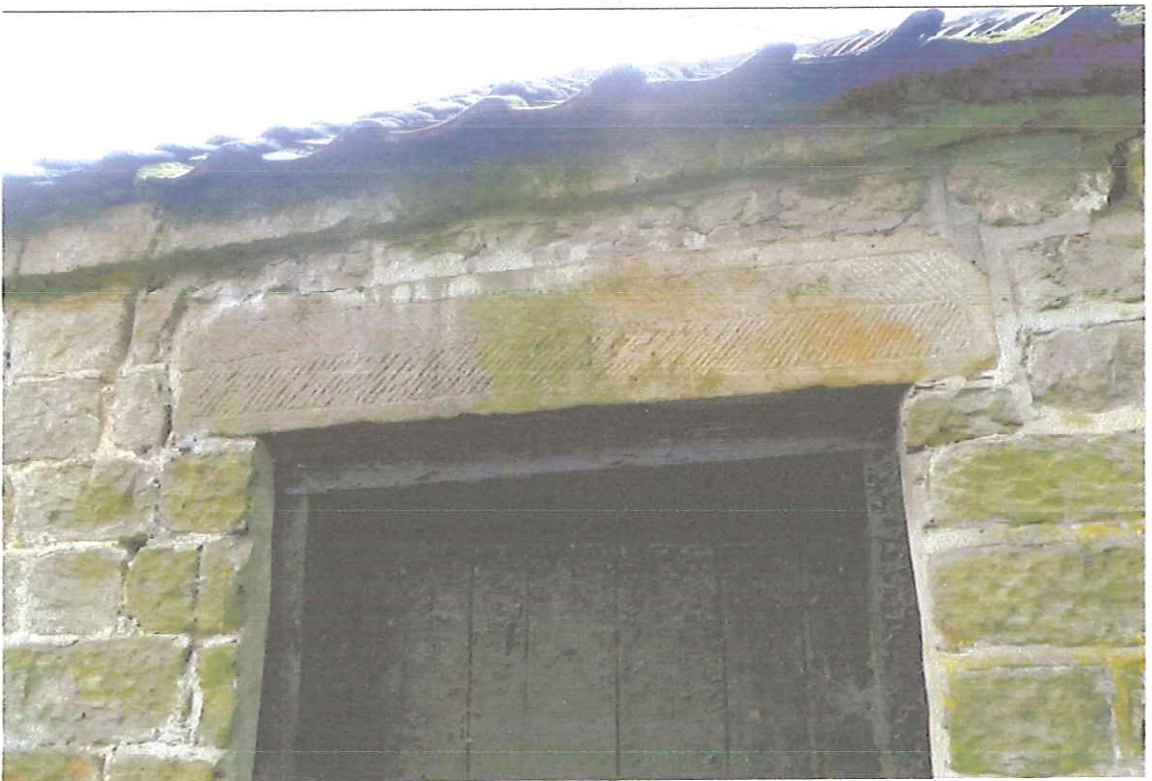
8. Troutdale Mill. Herringbone tooled lintel over door in south-east elevation.
