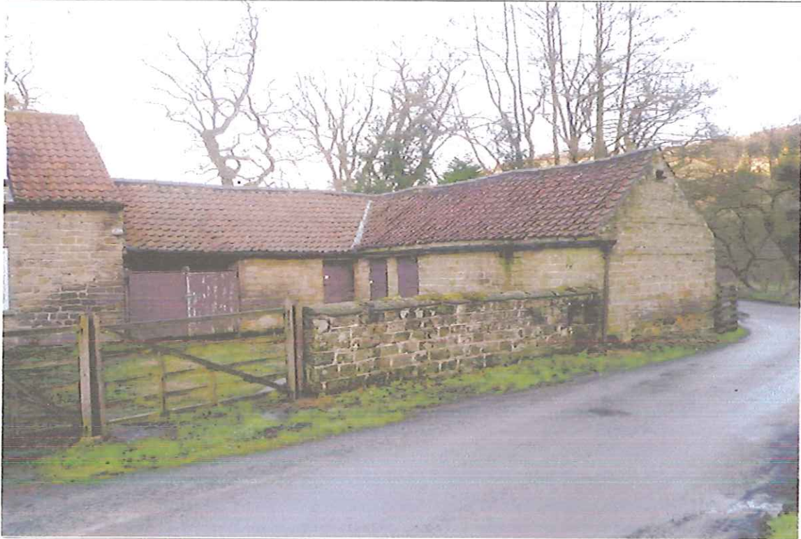
1. Troutsdale Mill. View of attached farm buildings from south west.
