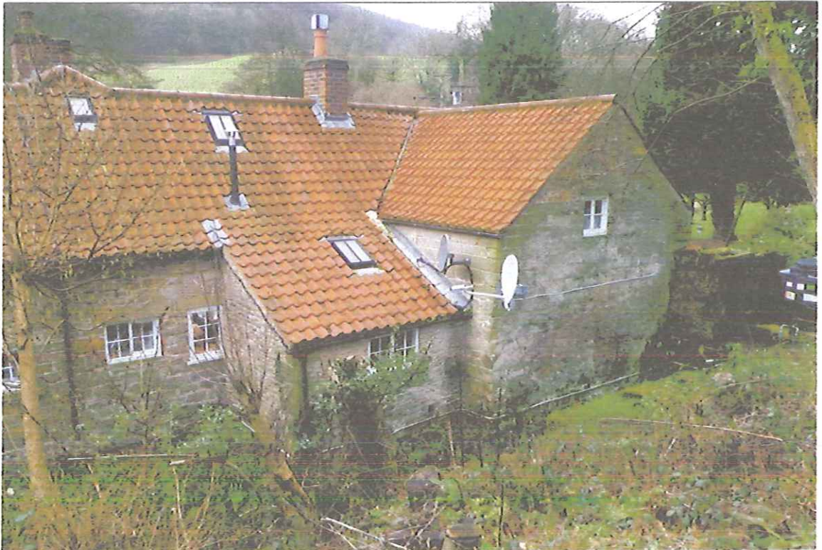
3. Troutdale Mill. North-east elevation of the mill house, with mill to the right. The stonework which supported the leat which fed the overshot wheel is to the right.
