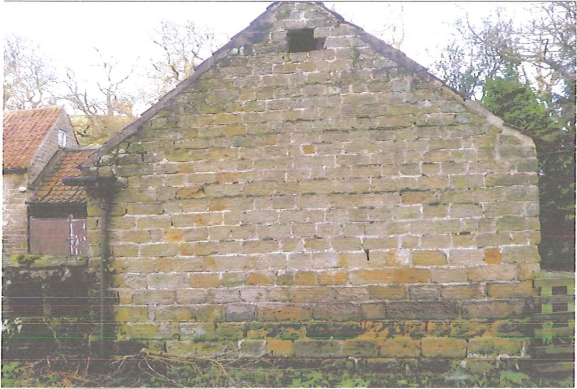
5. Troutsdale Mill. South gable end showing probable owl hole.
