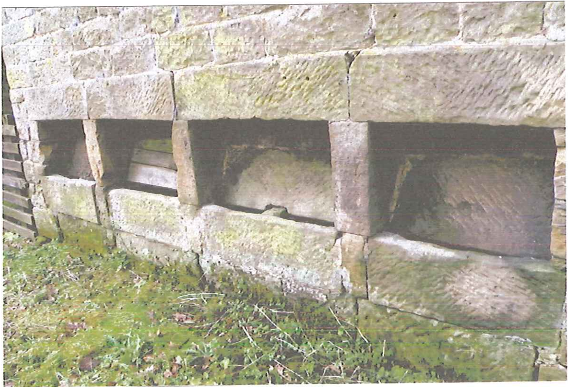
7. Troutdale Mill. Stone pig feeders in the south-east elevation.
