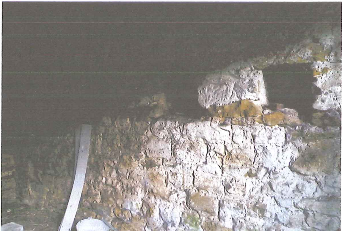
10. Troutsdale Mill. Niches in the south-east wall of Store 1, cart shed.
