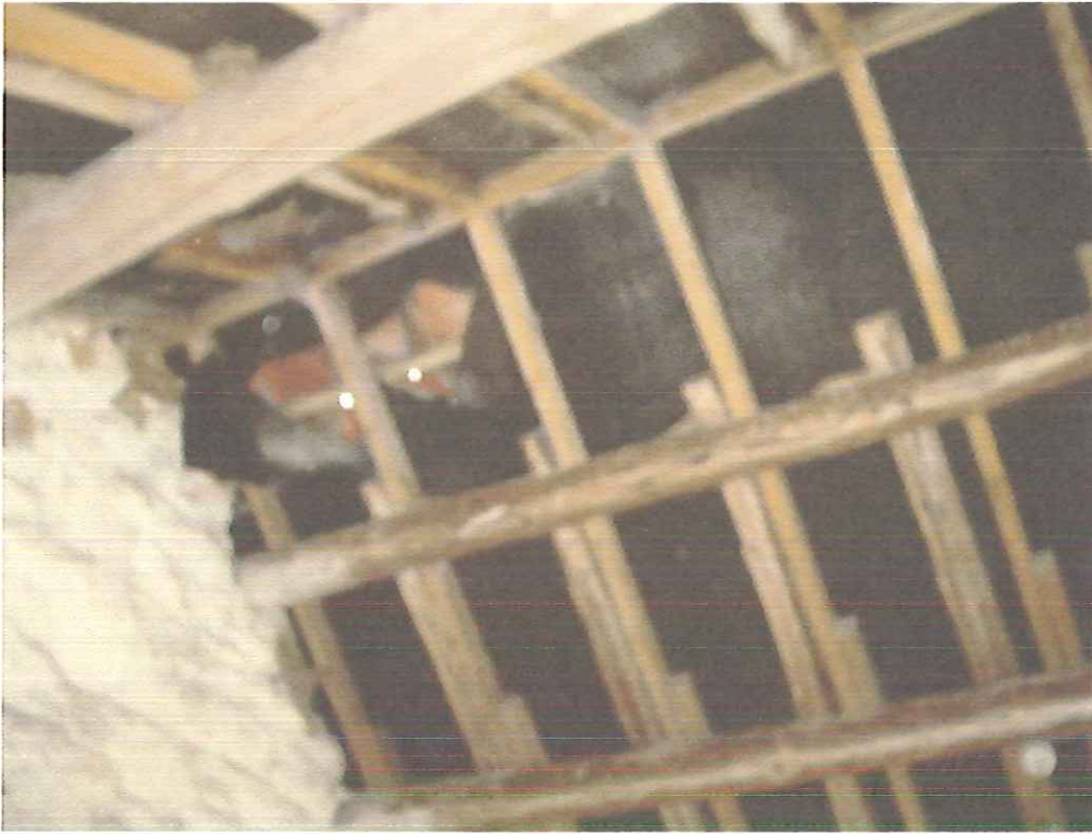
Figure 11 – ROOF-STORE 1 - NORTH SLOPE
