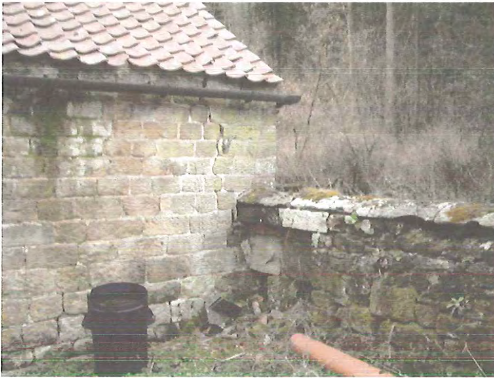
Figure 7 - COURT YARD LOOKING EAST
