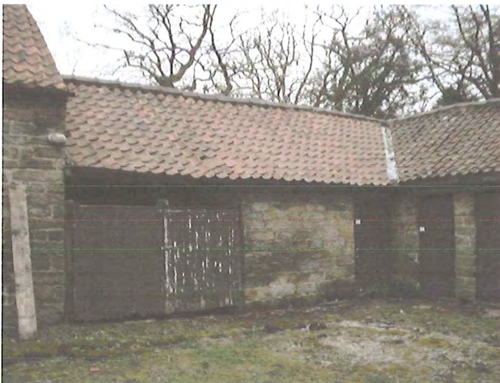
Figure 10 - COURT YARD LOOKING NORTH
