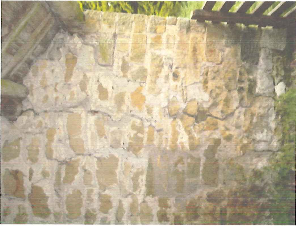
Figure 17 - STORE 5-NORTH WALL
