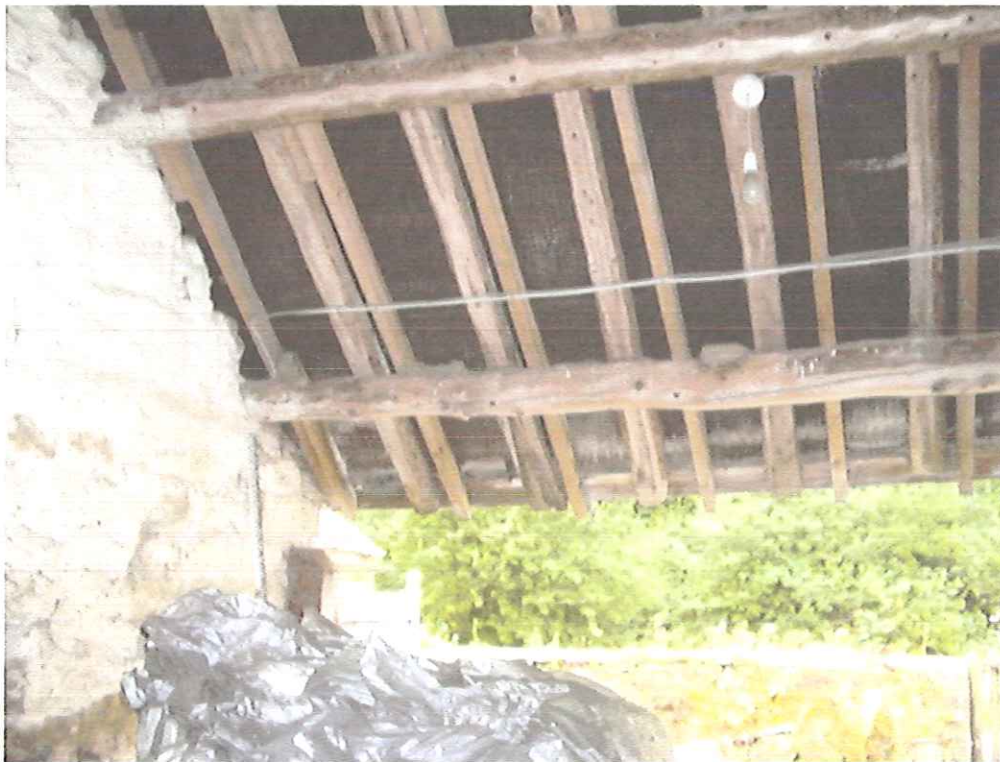
Figure 12 – ROOF-STORE 1-SOUTH SLOPE
