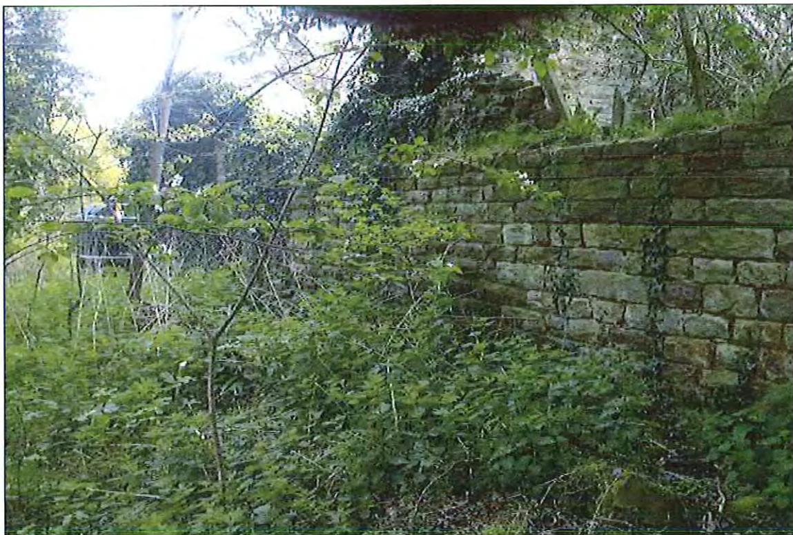
PHOTOGRAPH 6 Building D from the North
