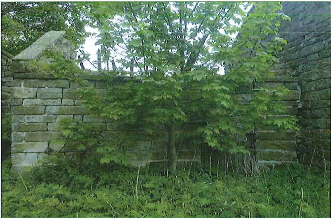
PHOTOGRAPH 4 Building B from the West
