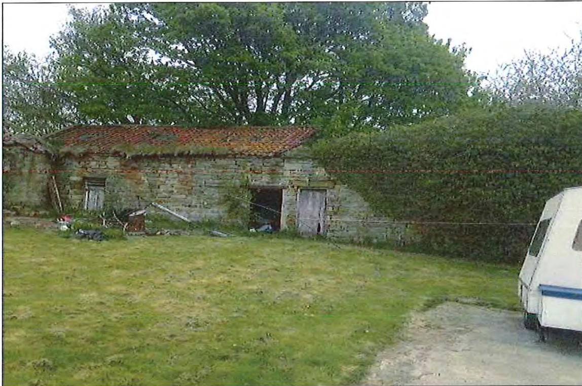
PHOTOGRAPH 1 Building D and C from the South
