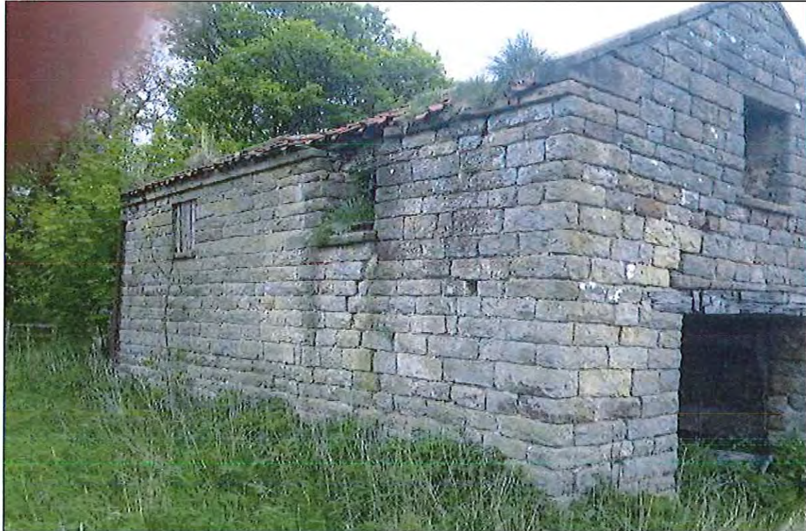
PHOTOGRAPH 3 Building A from the West
