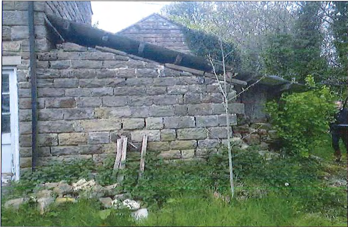
PHOTOGRAPH 7 Building E from the East
