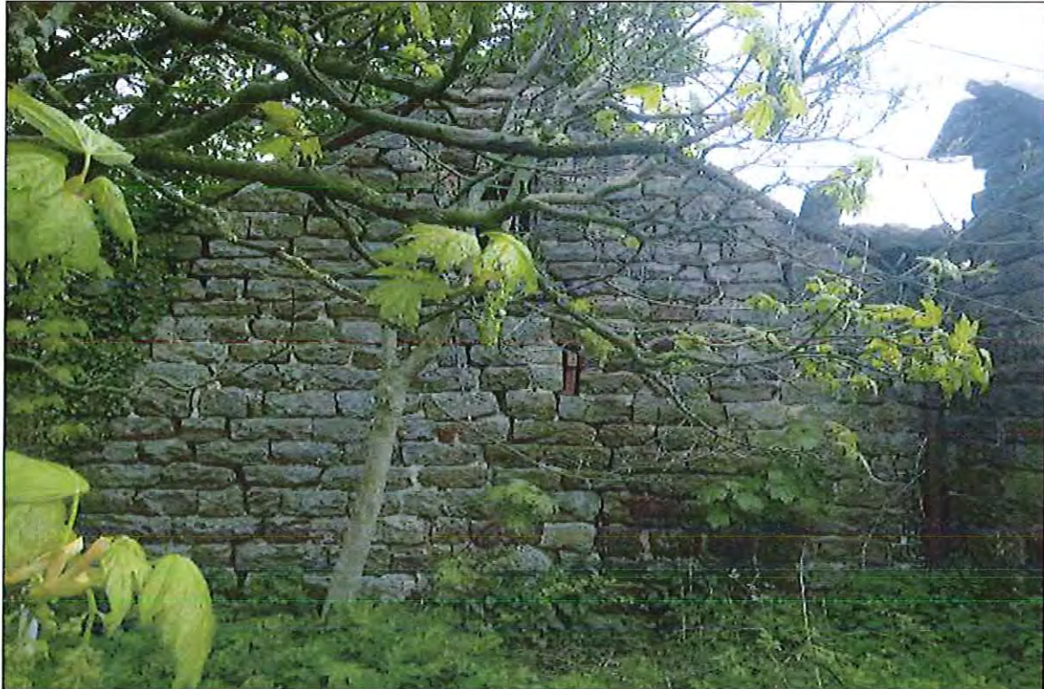
PHOTOGRAPH 15 CALFTHWAITE FARM, CLOUGH – BARN C
