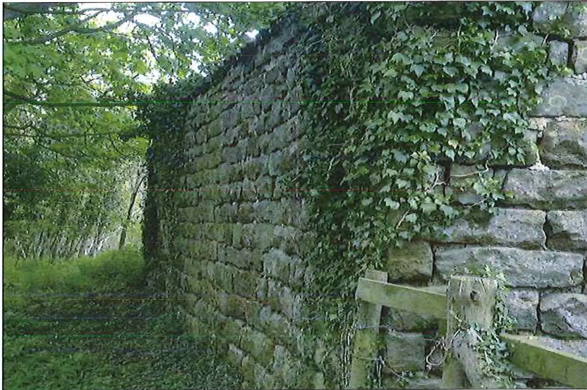
PHOTOGRAPH 17 CALFTHWAITE FARM, CLOUGH – BARN C
