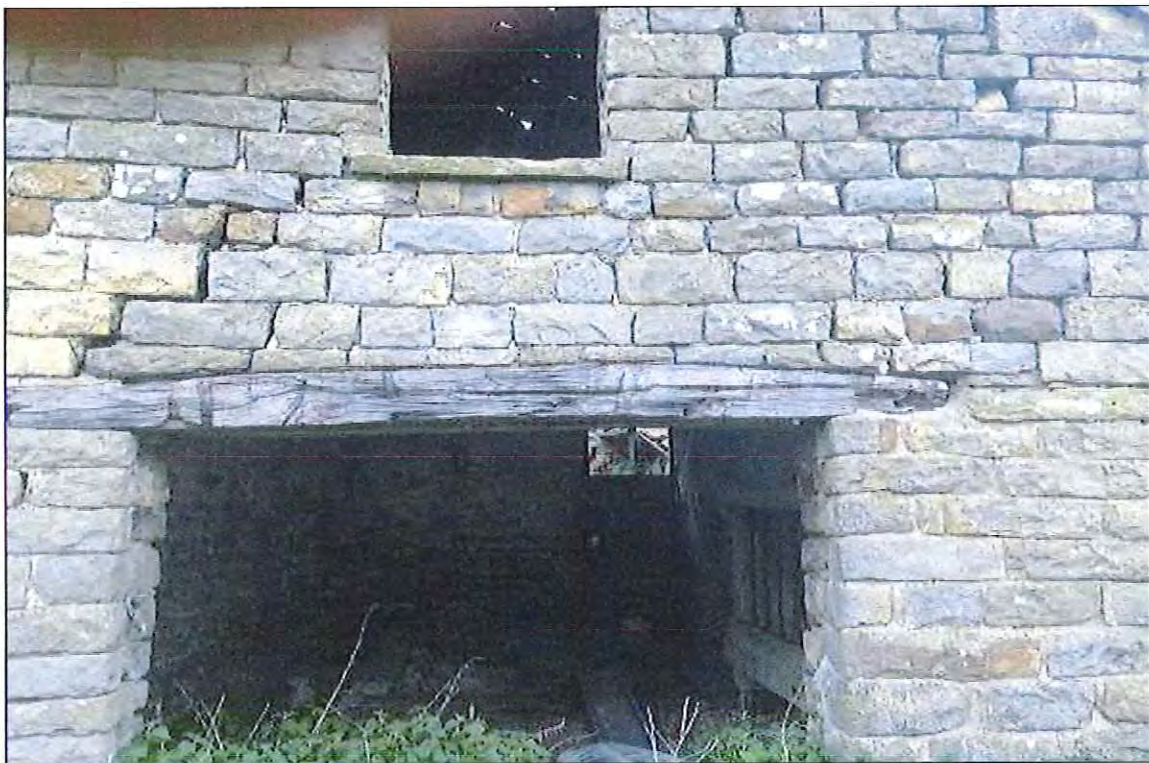
PHOTOGRAPH 4 CALFTHWAITE FARM, CLOUGH – BARN A
