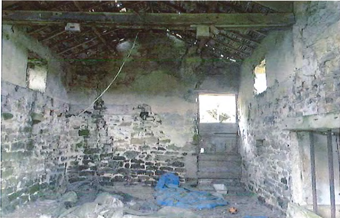
PHOTOGRAPH 7 CALFTHWAITE FARM, CLOUGH – BARN A
