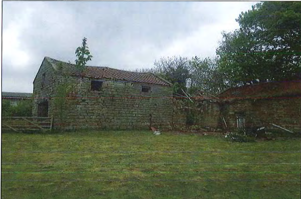
PHOTOGRAPH 1 CALFTHWAITE FARM, CLOUGH – BARN A
