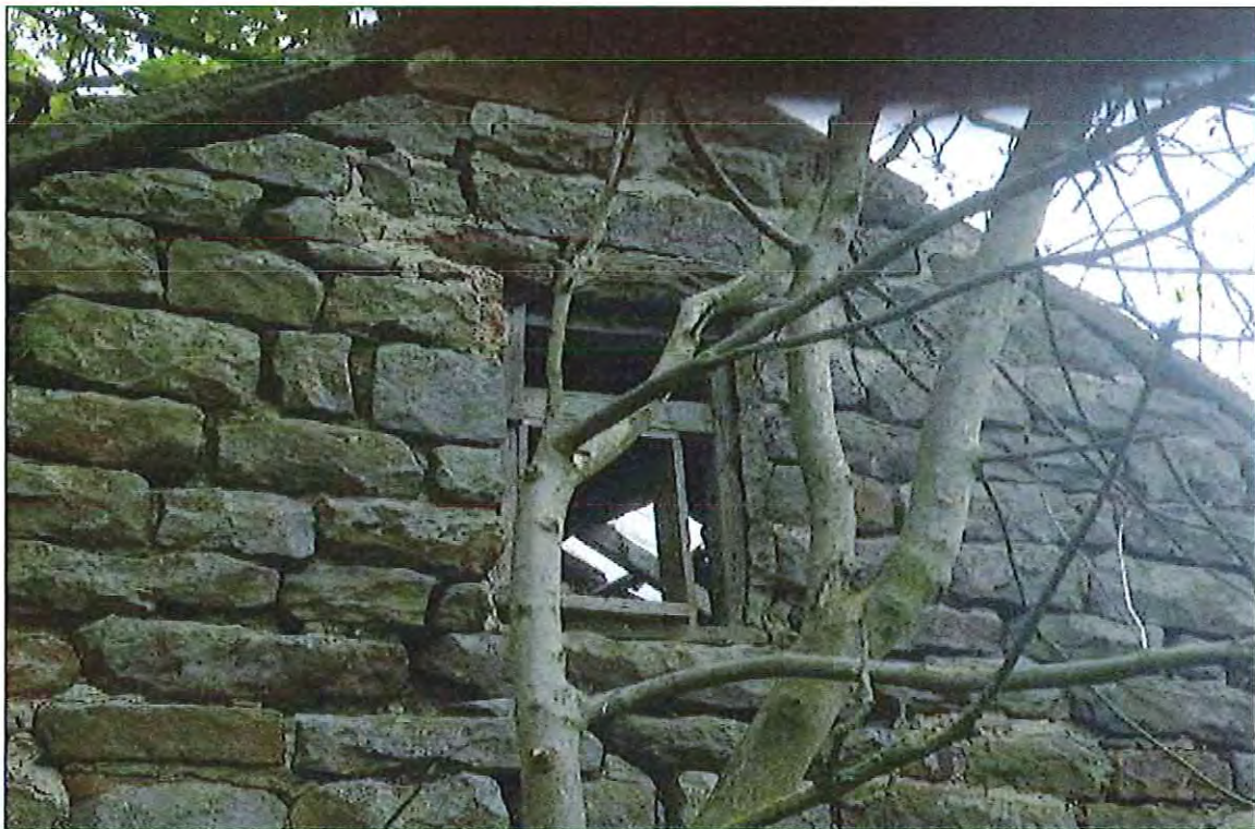
PHOTOGRAPH 16 CALFTHWAITE FARM, CLOUGH – BARN C
