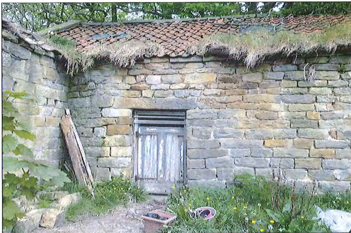
PHOTOGRAPH 14 CALFTHWAITE FARM, CLOUGH – BARN C
