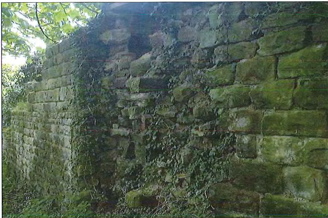
PHOTOGRAPH 18 CALFTHWAITE FARM, CLOUGH – BARN C
