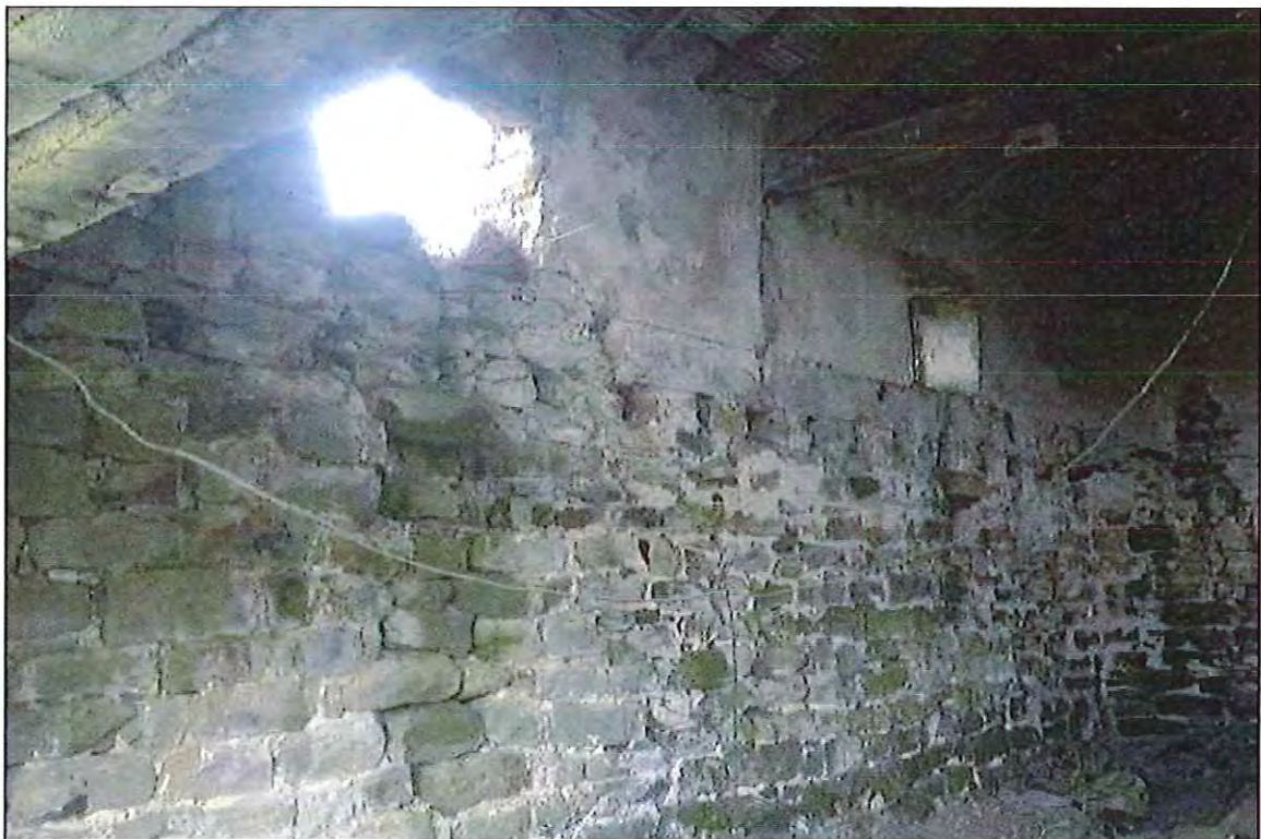
PHOTOGRAPH 8 CALFTHWAITE FARM, CLOUGH – BARN A
