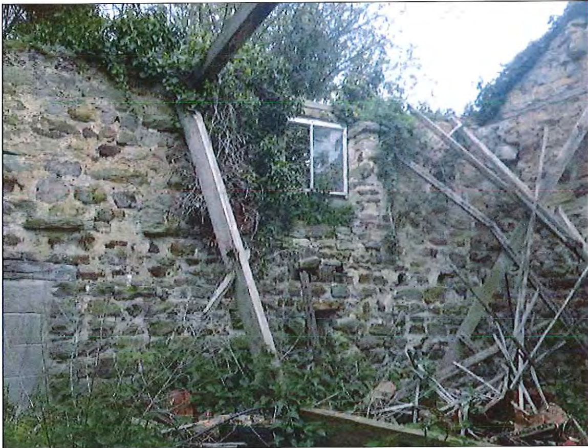
PHOTOGRAPH 26 CALFTHWAITE FARM, CLOUGH – BARN D
