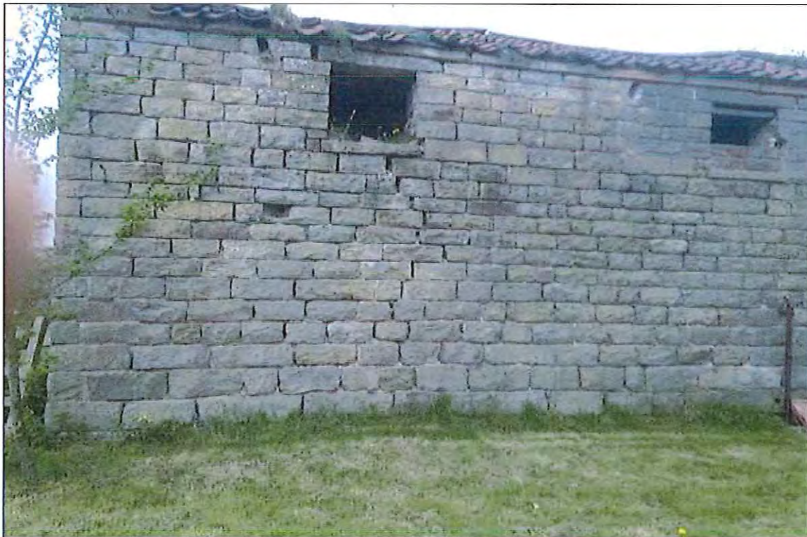
PHOTOGRAPH 2 CALFTHWAITE FARM, CLOUGH – BARN A
