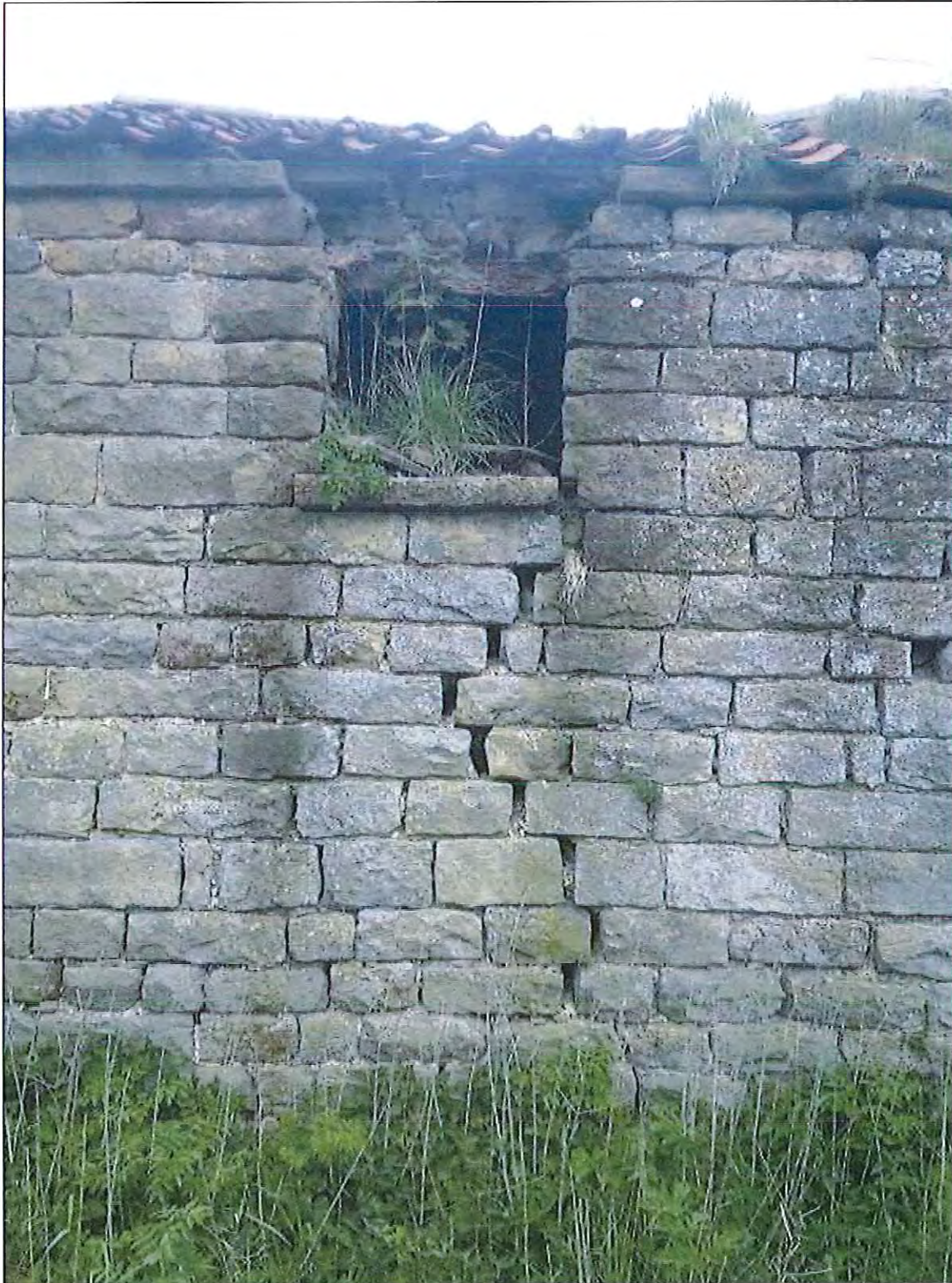
PHOTOGRAPH 6 CALFTHWAITE FARM, CLOUGH – BARN A
