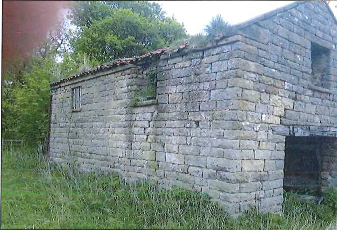
PHOTOGRAPH 5 CALFTHWAITE FARM, CLOUGH – BARN A
