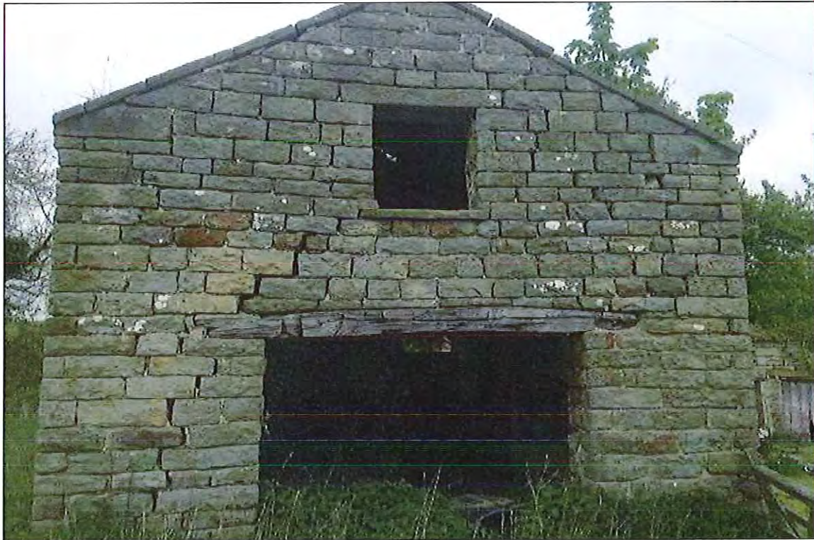
PHOTOGRAPH 3 CALFTHWAITE FARM, CLOUGH – BARN A
