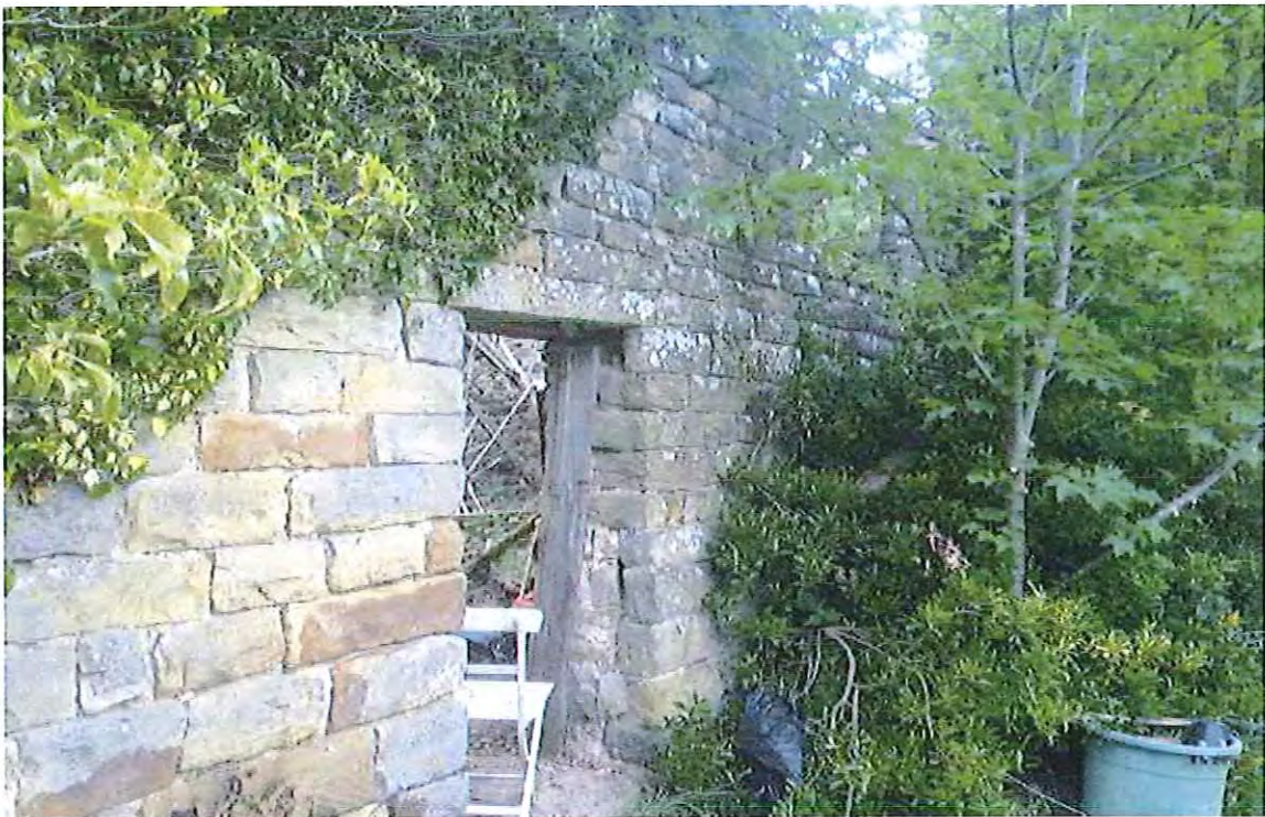
PHOTOGRAPH 22 CALFTHWAITE FARM, CLOUGH – BARN D
