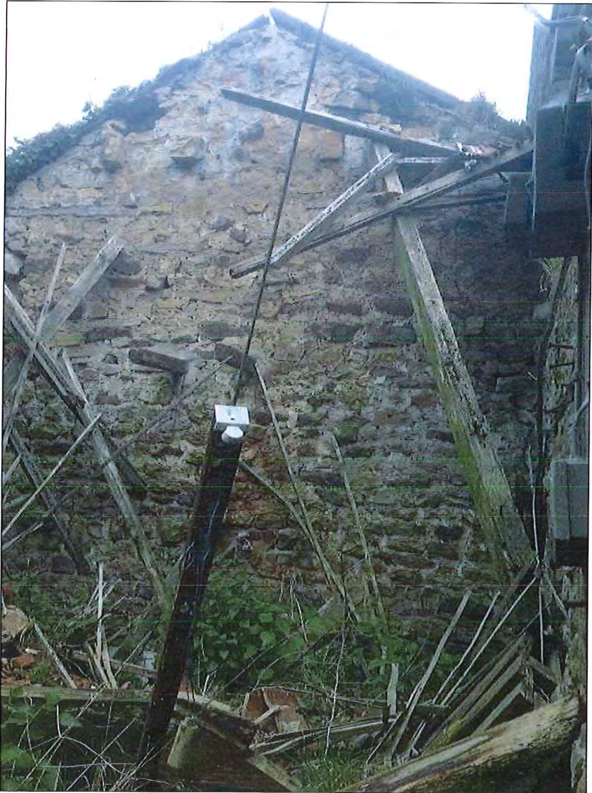
PHOTOGRAPH 25 CALFTHWAITE FARM, CLOUGH – BARN D
