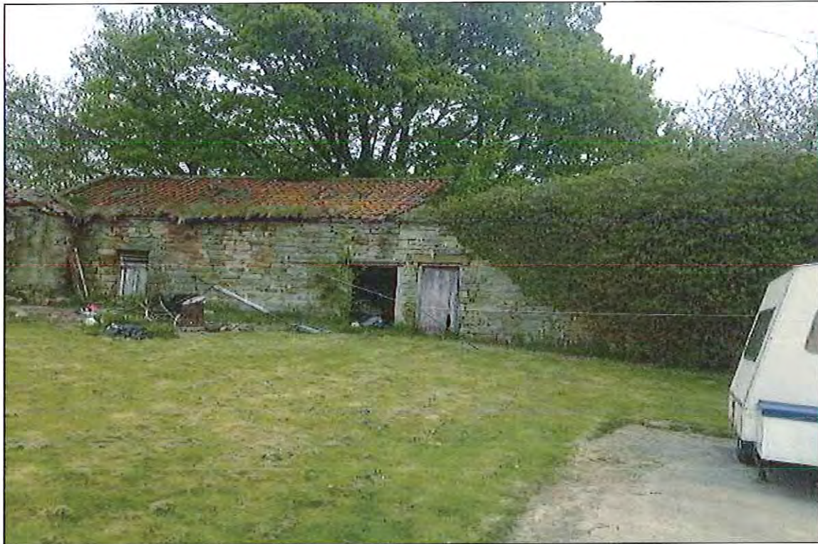
PHOTOGRAPH 13 CALFTHWAITE FARM, CLOUGH – BARN C
