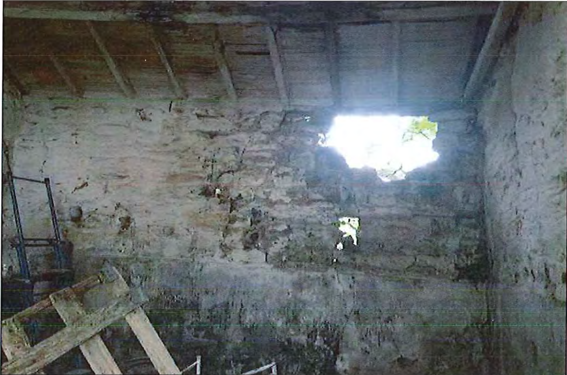
PHOTOGRAPH 19 CALFTHWAITE FARM, CLOUGH – BARN C
