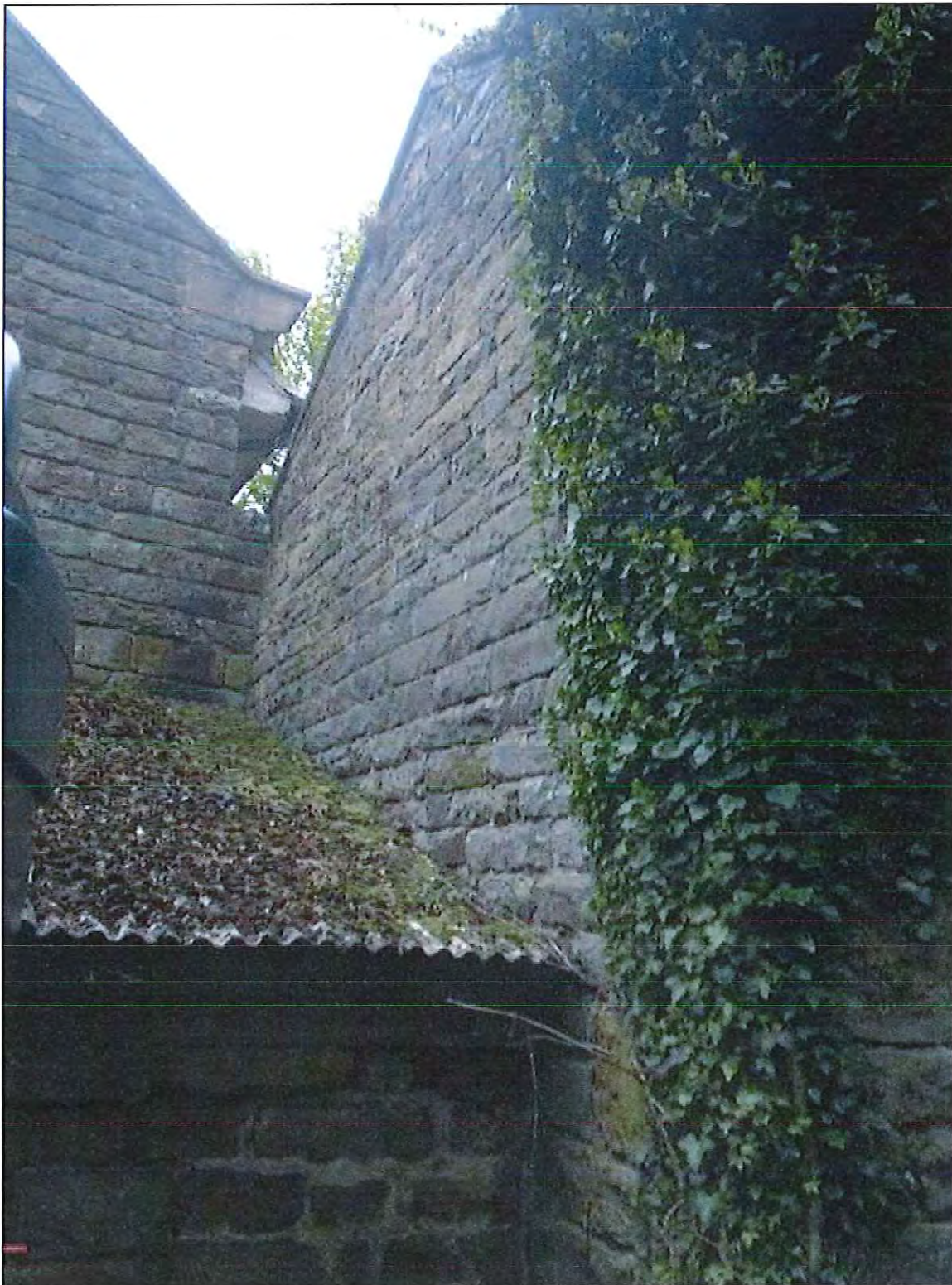
PHOTOGRAPH 24 CALFTHWAITE FARM, CLOUGH – BARN D
