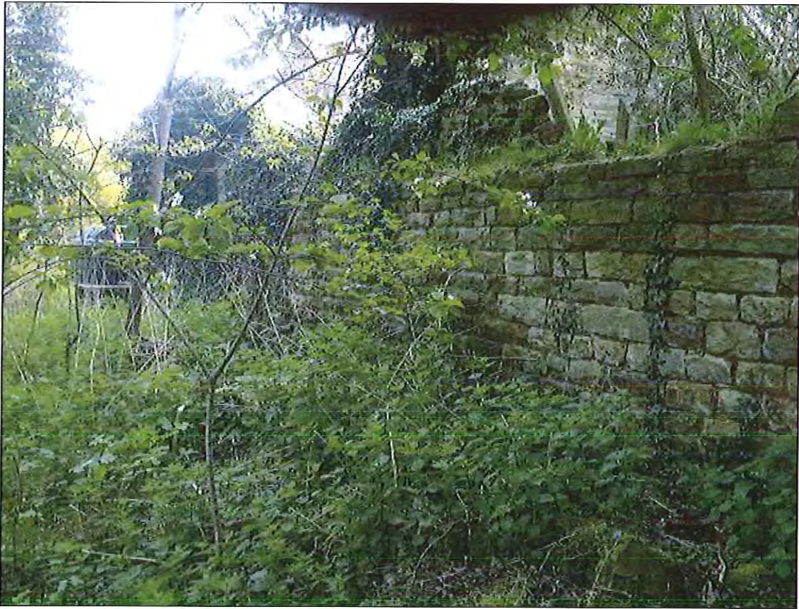
PHOTOGRAPH 23 CALFTHWAITE FARM, CLOUGH – BARN D
