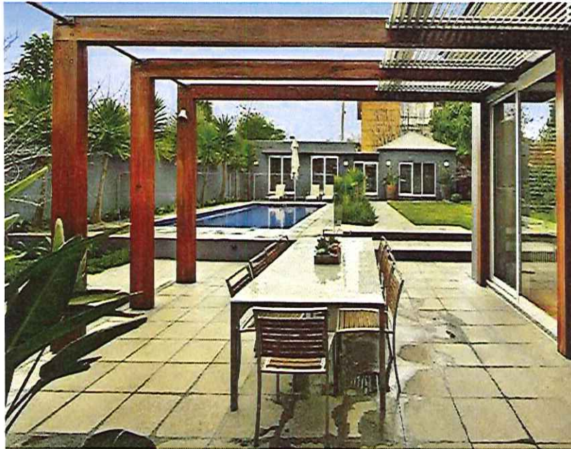
Pergola structure above decking to carry sails
