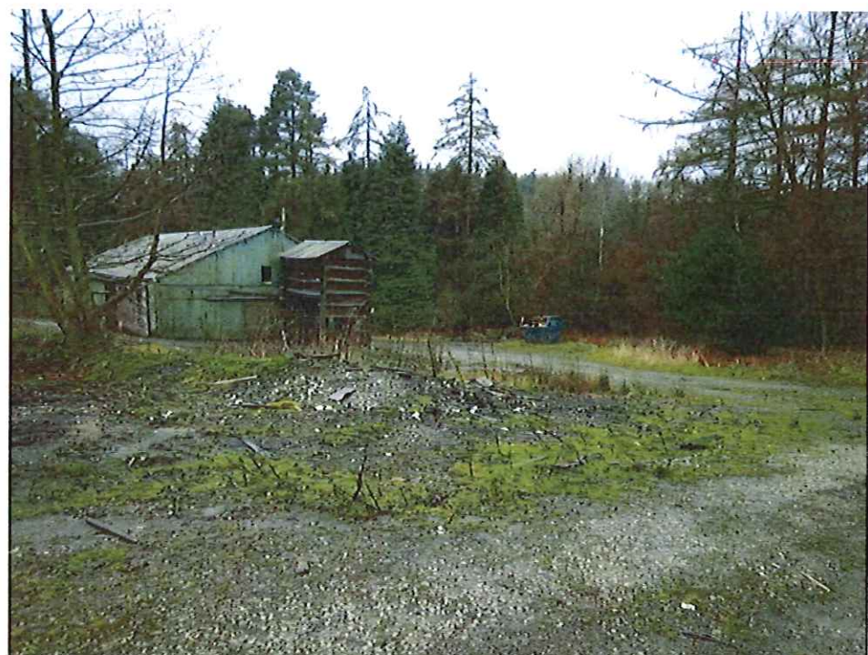
Photograph 10. Areas of hard standing to the north and west of the saw mill. The wooden sawdust storage tower can be seen on the north side of the saw mill.
