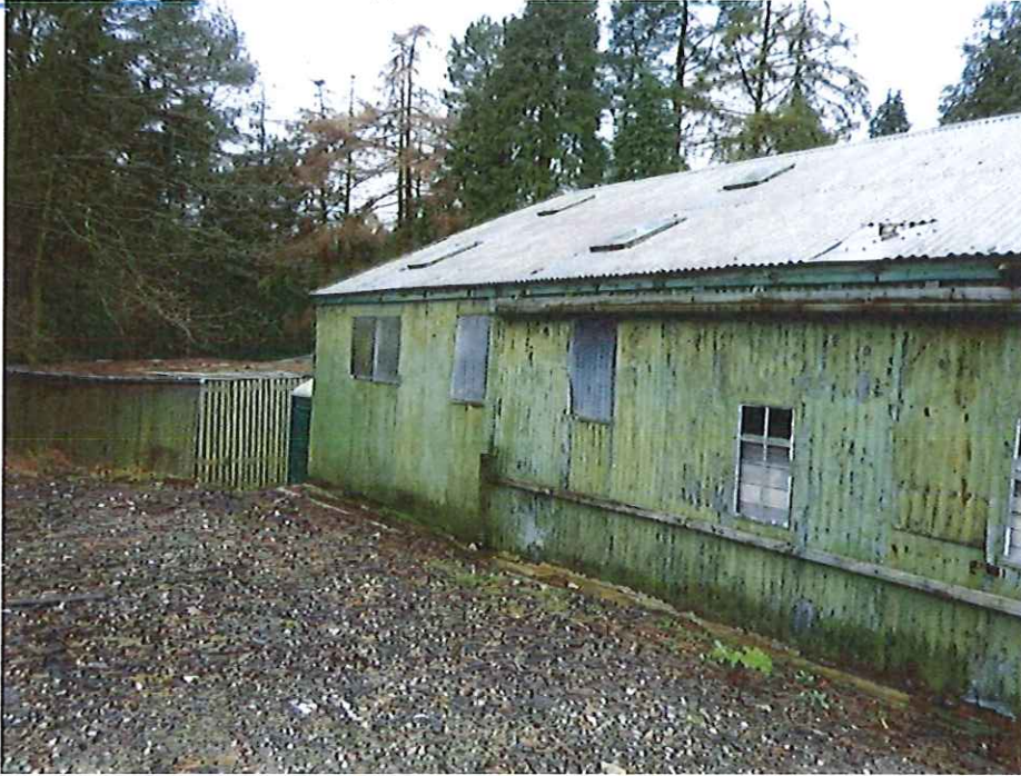
Photograph 1. Exterior of the saw mill with building 1 in the background
