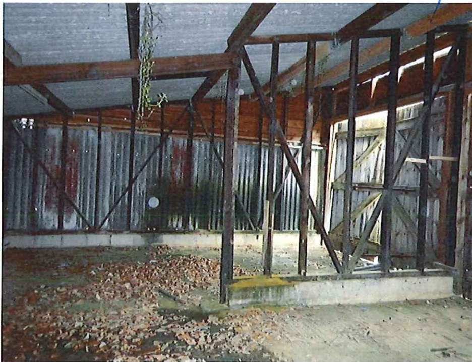
Photograph 7. Interior of the northern end of building 3
