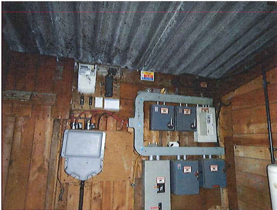
Photograph 4. Interior of the switch room
