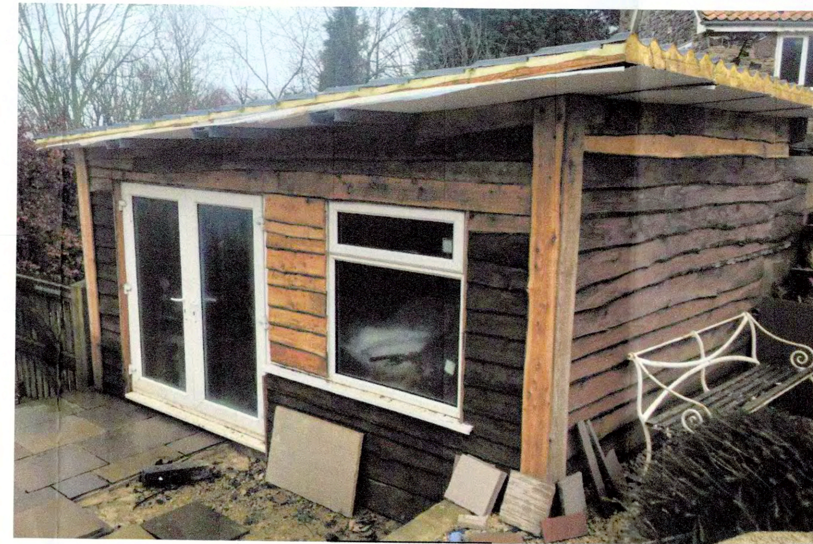
NORTH WEST VIEW
