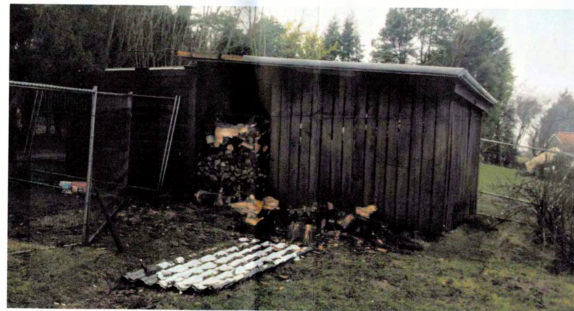
LOG STORE NORTH VIEW
