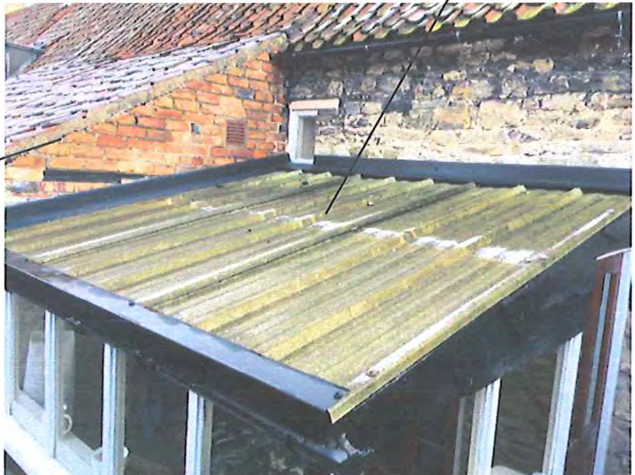
replacement pantiled roof to be raised to same level as existing roof over kitchen
