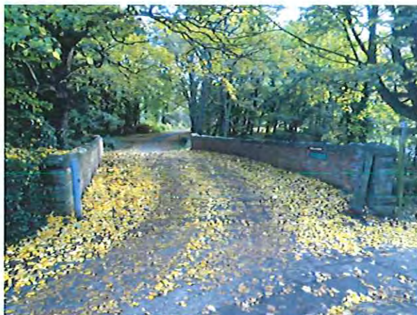
Access to the site from Lowdale Lane within Sleights village
