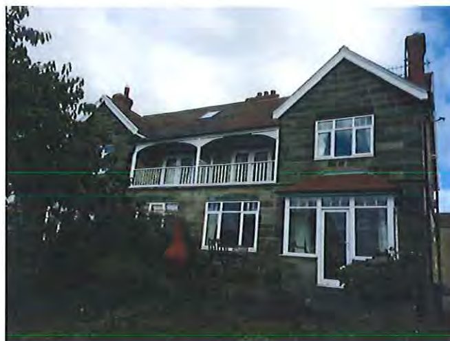
Western façade of 4 Echo Hill facing Sleights village
