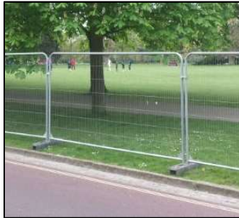
2m tall anti-climb fencing
