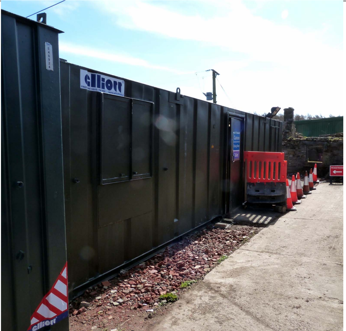
Office Container, typical
