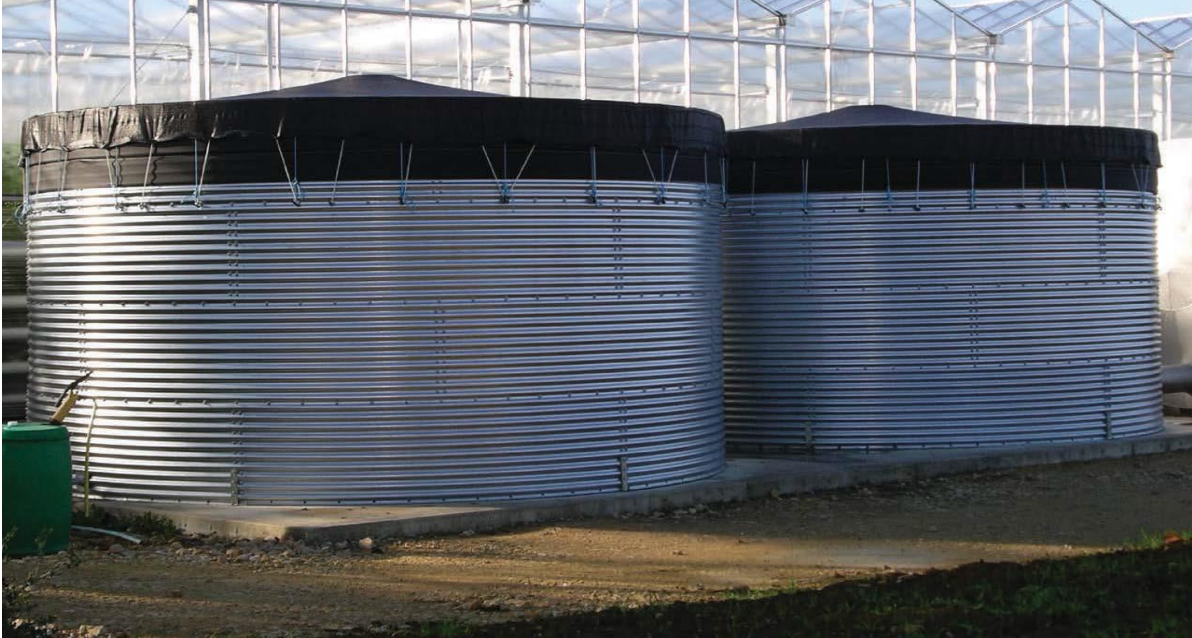
Photograph 3 – Typical water tanks associated with the concrete batching plant
