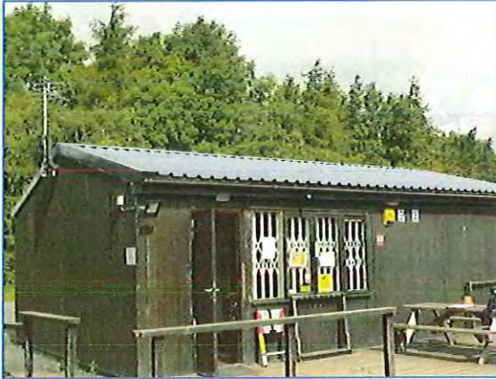
Photo 2: Building from south east.
