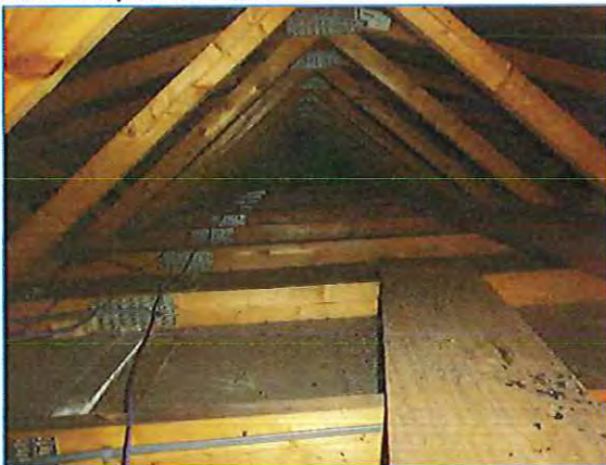
Photo 6: Cluttered roof void.
