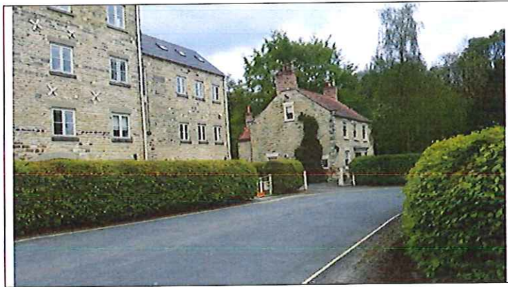
Photograph showing the relationship of the Mill to the Mill House.
