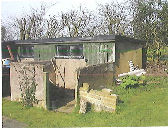
Front elevation from adjacent wall.
