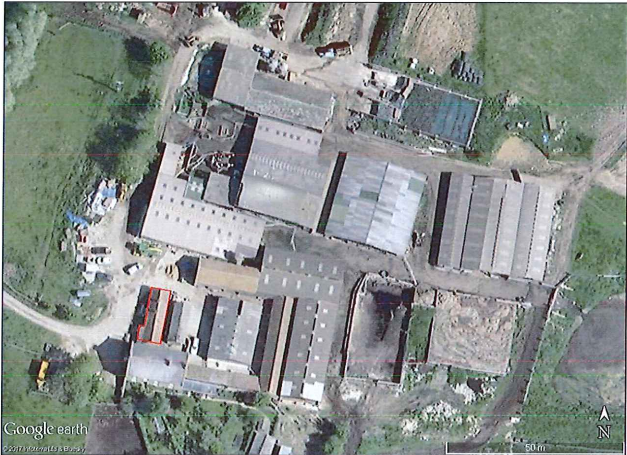
Figure 2: Aerial view of Burgate Farm with surveyed building outlined
