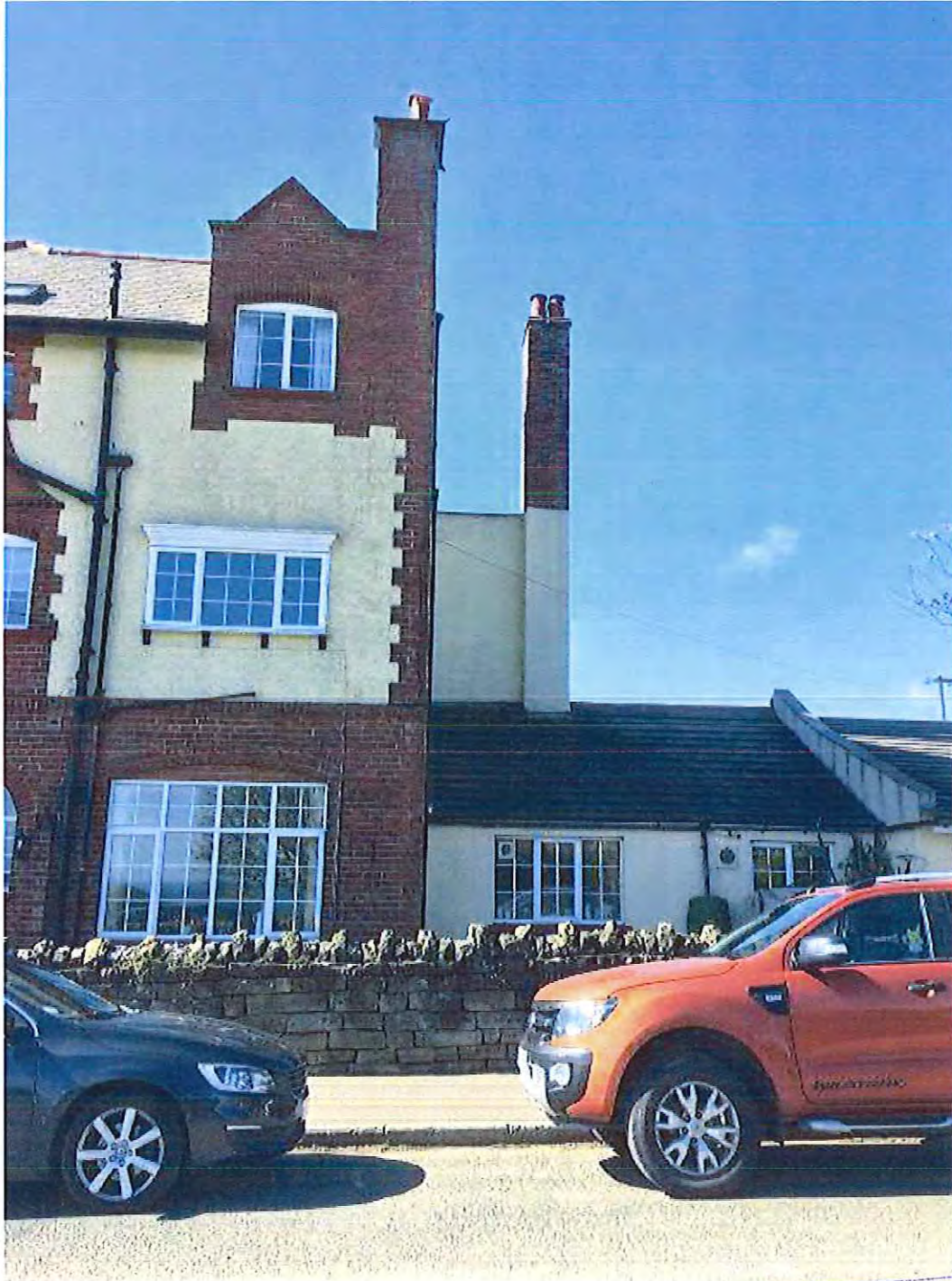
Picture 1 Part main Building, Part Lean-to
