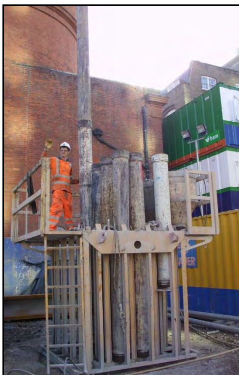
Figure 9: Photo of tremie string assembly
