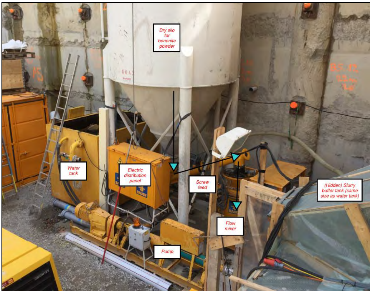
Figure 1: Typical slurry mixing setup
