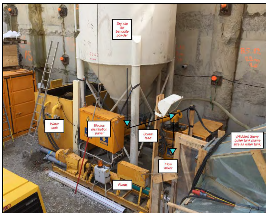
Figure 5: Typical slurry mixing setup
