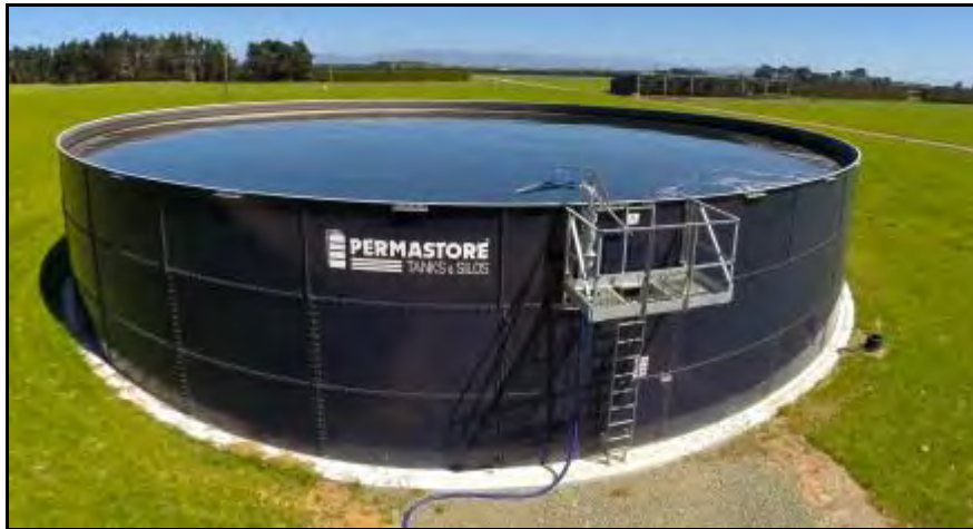
Figure 2: Photograph of typical storage tank
