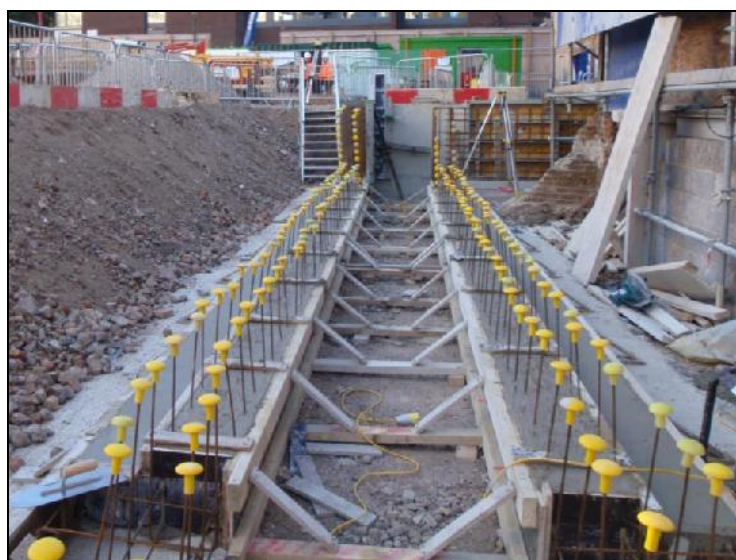
Figure 3: Construction of the base
